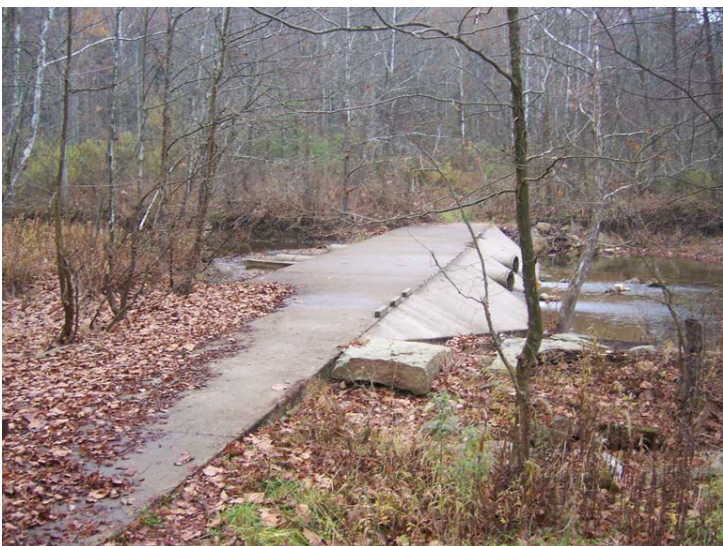
One of two culvert bridges to be removed
