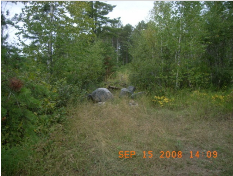
Figure 14.2 One year (2008) after decommissioning a road on the Nira Project 13 on the Superior National Forest.
