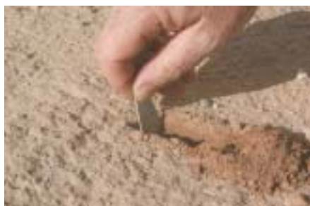
Figure 13. Excavate small trench.
