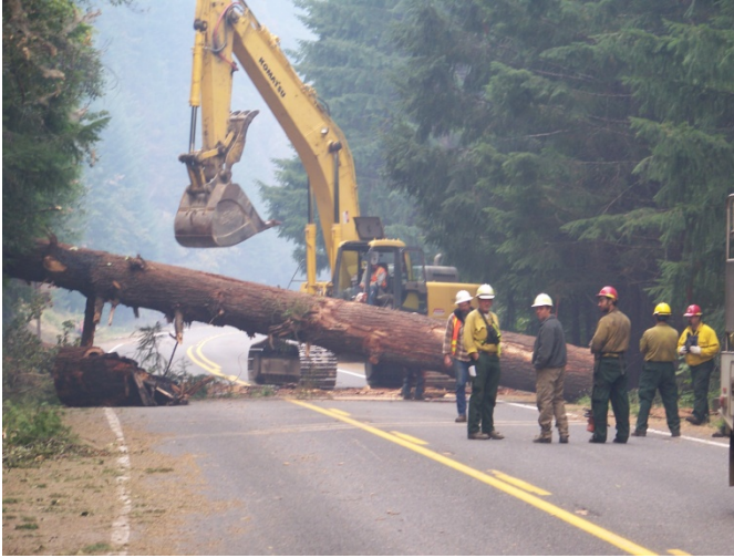
ODOT removing trees from Highway 138 with a trackhoe
