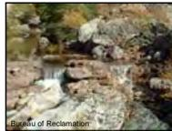
A fish barrier was constructed in 2004 upstream of the Verde River. This small structure is not a dam, but allows the natural flow of water while preventing non-native fish from moving further upstream into Fossil Creek. Non-native fish are a serious threat to native fish in Arizona.
