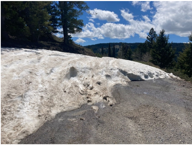
Snow drift blocking Sinks road 5/26/2021.
