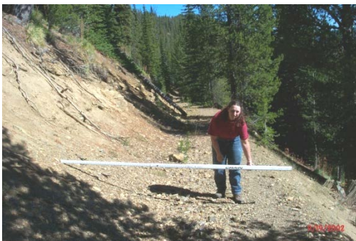
Old road that would be authorized for motorized access within the FC-RONR Wilderness.
