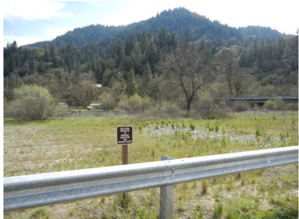
Photo 3 (After): This picture was taken from about the same spot as the first one (The bridge over the West Fork can be seen in the background), about 2 years after completion. Native vegetation has been established creating a bio-filter for overland flow coming from the remaining riding area.
