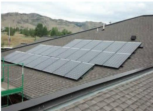
6 kilowatt solar photovoltaic system at the Boulder Ranger District.
