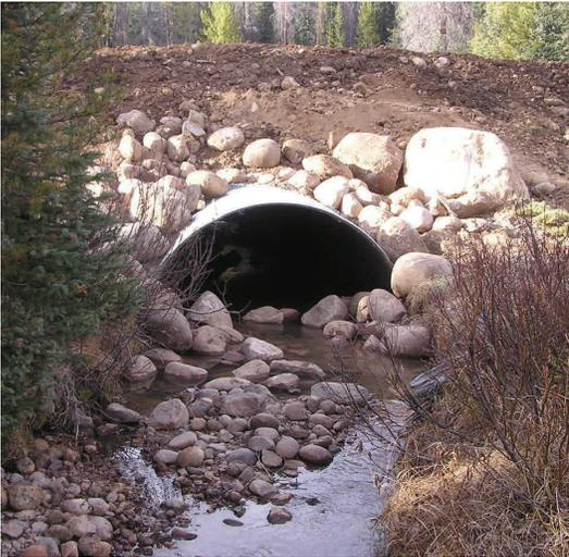
Forest Engineers helped with the design and installation of bottomless culverts. This project restored access to 2.5 miles of stream for native cutthroat trout in Trail Creek on the Sulphur Ranger District.
