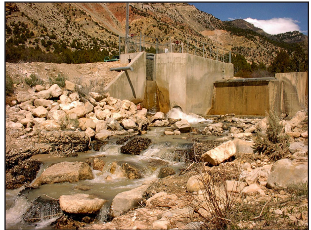
Figure 1. The bypass reach immediately below the Manti City Lower Power Plant diversion facility. The diversion partially dewateres about 1.5 miles of Manti Creek.
