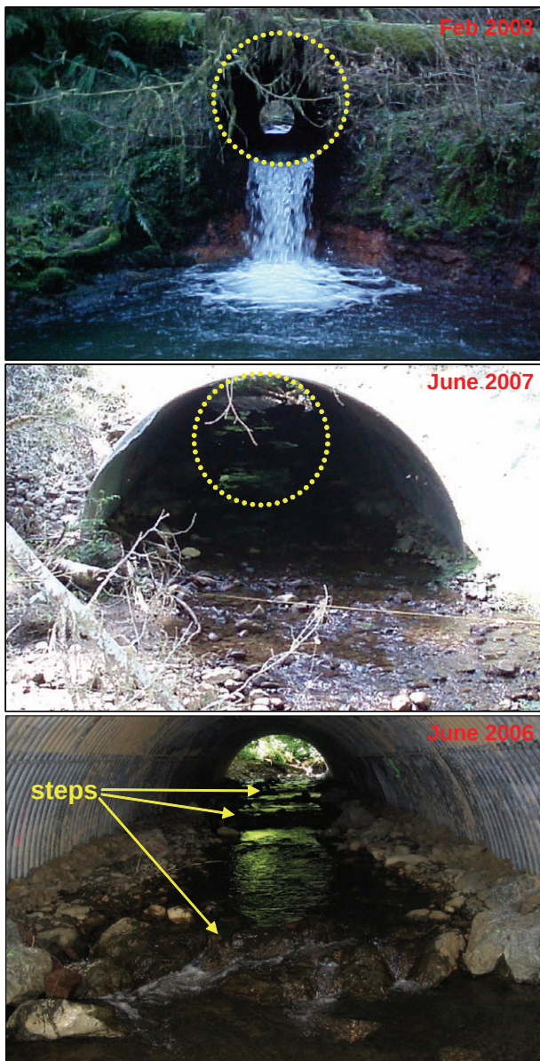
Figure 1. The replacement of the road-stream crossing structure on a tributary to the Middle Fork Salmon River (Olympic National Forest, Washington) using the stream-simulation approach. Upper Photo: Upstream view of the culvert outlet prior to replacement. The culvert was installed in the late 1950's, has a diameter of 1.83 m, a length of 27 m, and a gradient of 2.1 percent. The culvert outlet is perched 1.6 m above the pool. Middle Photo: Upstream view of the culvert outlet after the existing structure was replaced in October 2005. The open-bottom arch has a span of 5.49 m, a height of 2.25 m, a length of 29 m, and channel gradient of 4.1 percent. Lower Photo: The channel bed design through the structure contains a sequence of steps and pools, providing geomorphic continuity between the upstream and downstream channel.
