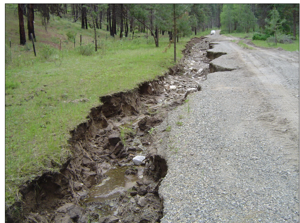
Figure 2. Washed out ditch. The ditch could not accommodate the increased post-fire flow.
