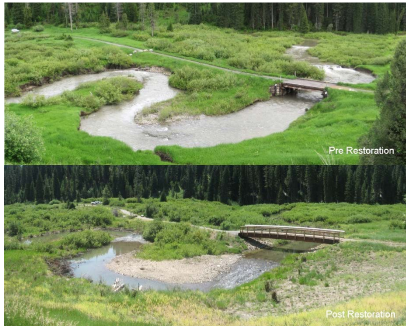
Figure 3: Jackknife Creek road bridge replacement and conversion to a wider-span, non-motorized trail crossing. Before and after restoration photos are provided.
