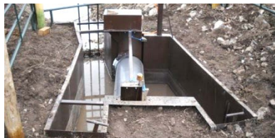
Figure 5: Solar-driven drum screen installed on the Jackknife Creek diversion. Viewed up ditch line, with a fish bypass pipe on the lower left and the ditch pipeline entrance on the lower right.
