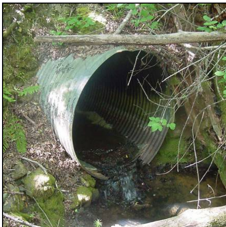
Existing Culvert Outlet
