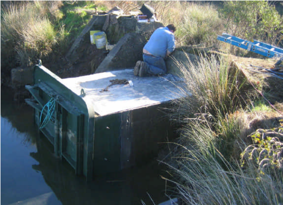
Figure 6. Installation of the aluminum ceiling to fully enclose the wing-walls to form a box culvert type structure.
