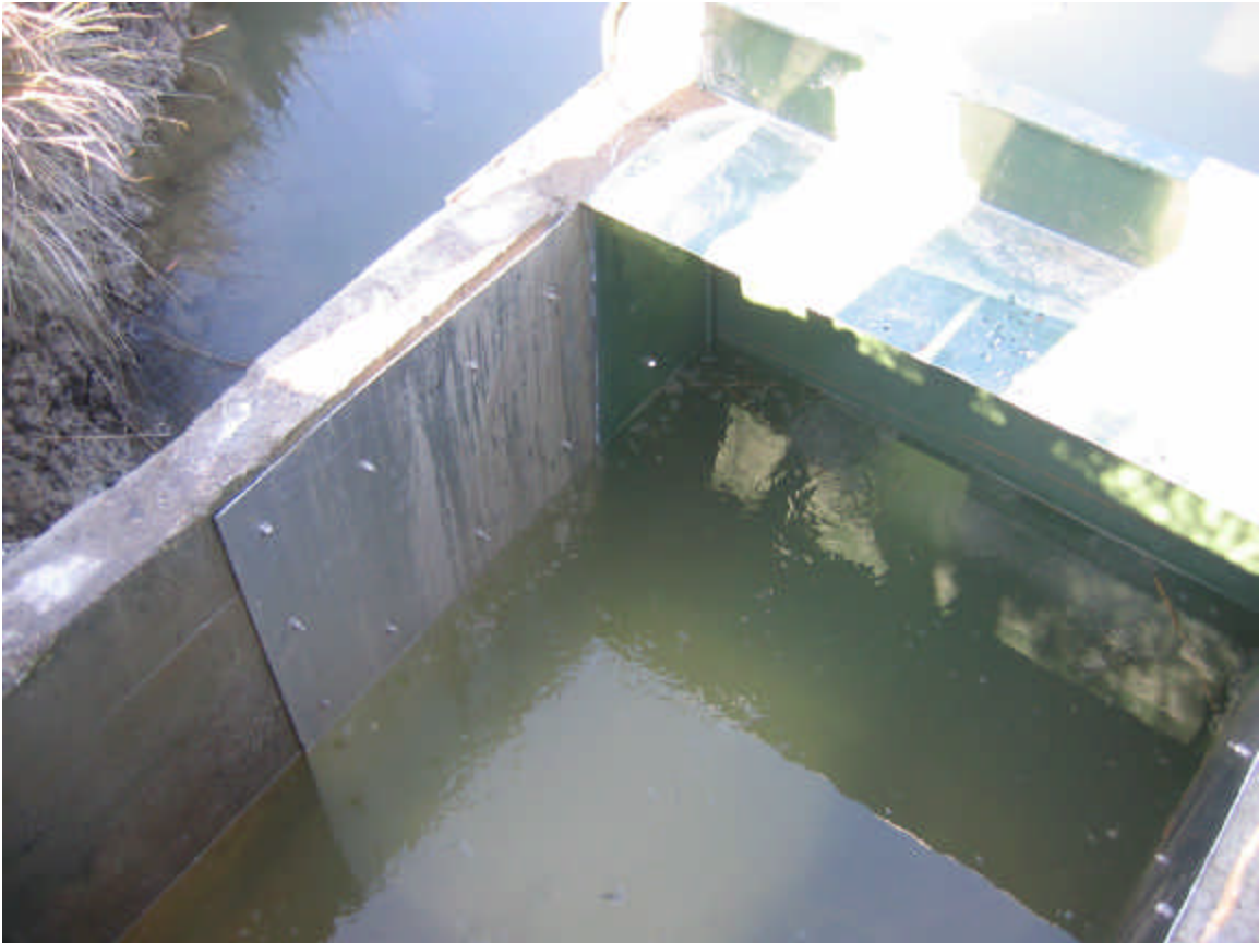
Figure 5. Top view of the new tidegate structure during assembly, before the aluminum ceiling was installed. The aluminum sleeves are shown bolted to the concrete wing-walls.
