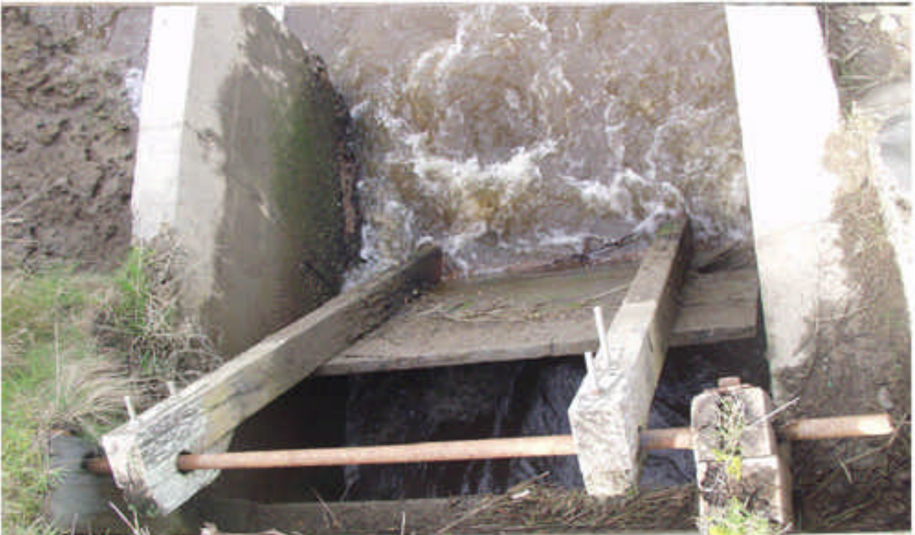
Figure 2. The old wooden tidegate on Rocky Gulch, at ebb tide. The top photo shows the abandoned tidegate to the left of the functioning tidegate.
