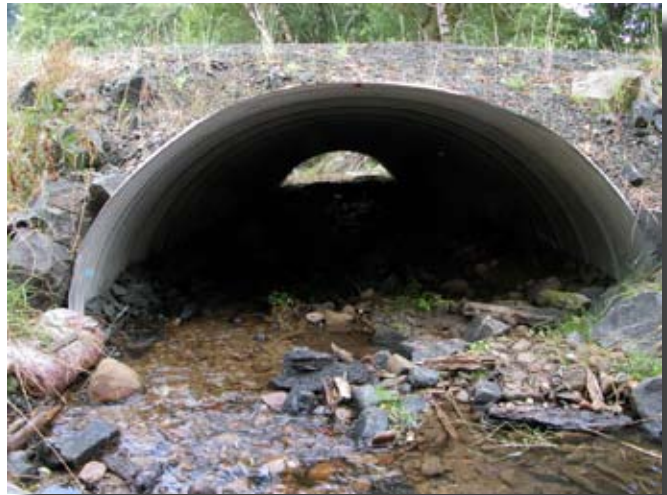
Figure 7.3—1-piece corrugated metal pipe arch (embedded).
