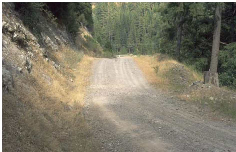
Figure 7.20—Diversion-prevention dip on the Plumas National Forest, California. The diversion dip is located just down the road from the stream crossing because the crossing is on a tight curve.
