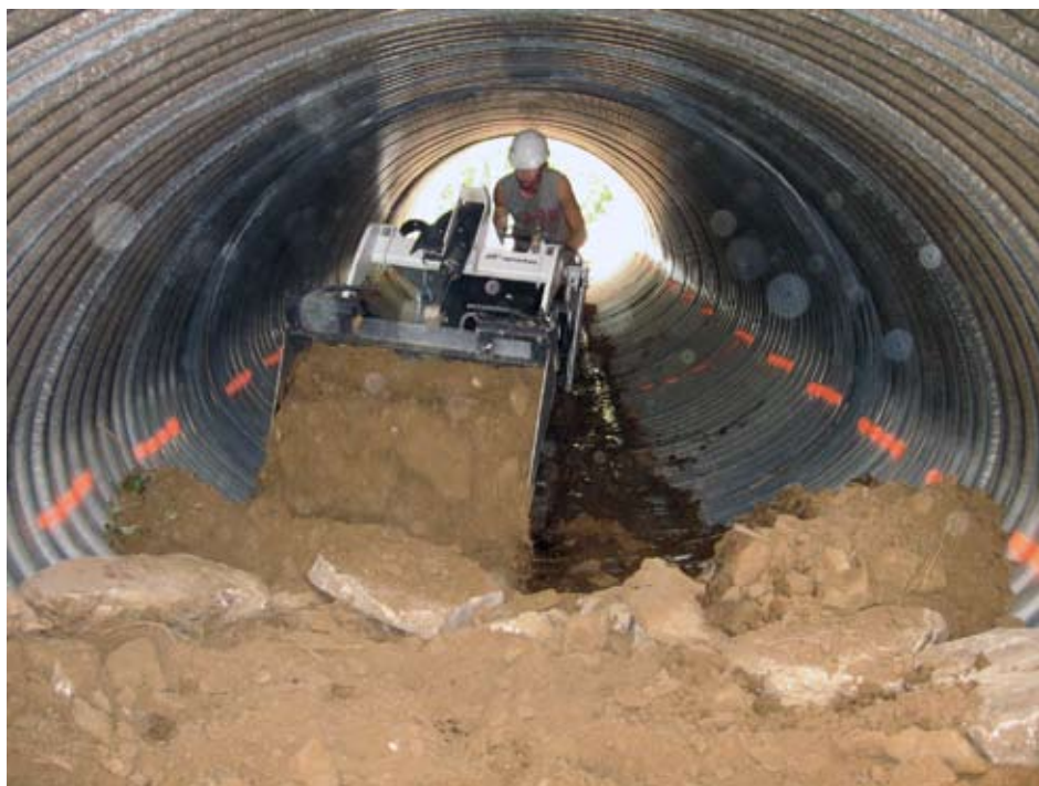
Figure 8.15—Bobcat placing bed material to marked elevation.
