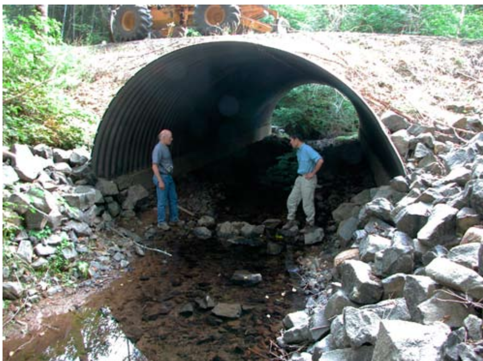
Figure 8.11—Example of uneven backfill and compaction. The right side was backfilled before the left side instead of even lifts on both sides, causing the distortion visible in this photo. The distortion induces eccentric loadings on the footings, as well as bending stresses at the anchor bolts on both footings.
