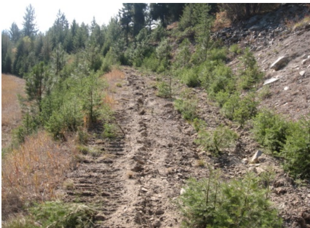
Example of road prism after decompaction with excavator & subsoiling grapple rack.
