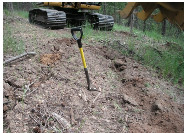
Sharpshooter shovel easily penetrated the previously compacted road bed after subsoiling was completed.
