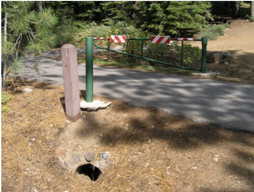
Figure 1-7. Camping spurs and the roadway were constructed over the top of the ephemeral stream using culverts in 8 locations on the site (indicated as stars on Figure 4).
