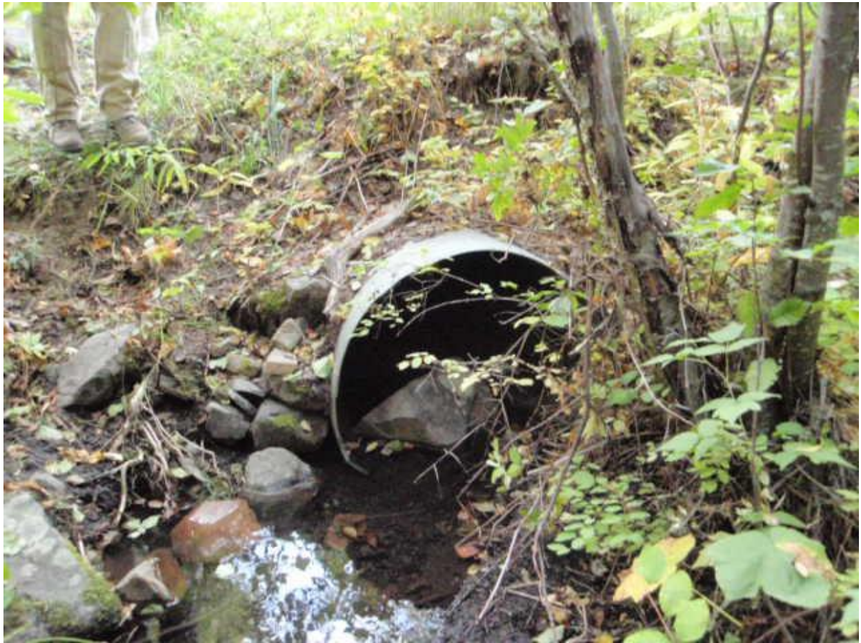
Figure 6 - FS Road 5515 crossing of Cromwell Creek.
