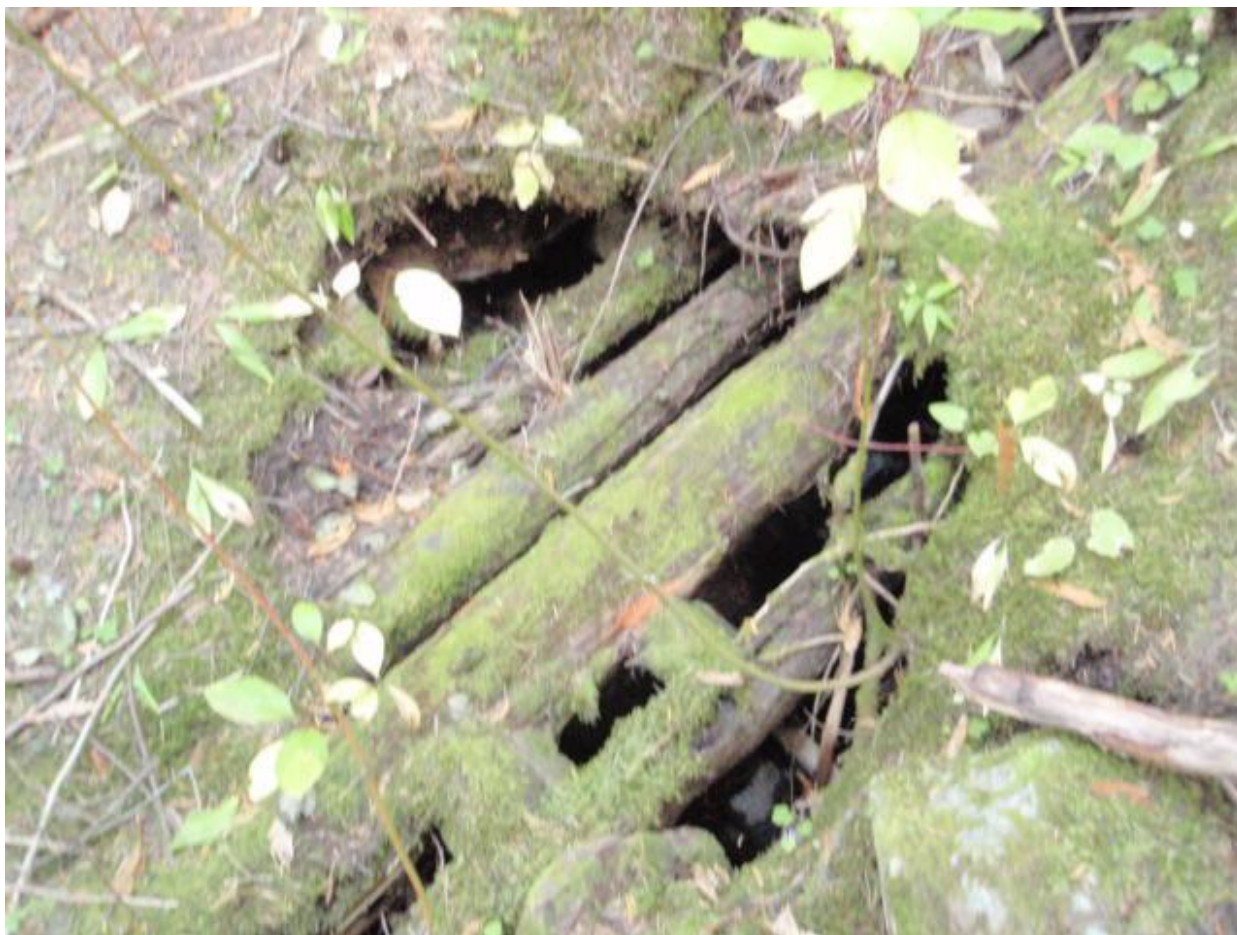
Figure 7. - Looking down on channel bed of Cromwell Creek and remnants of “corduroy road”.
