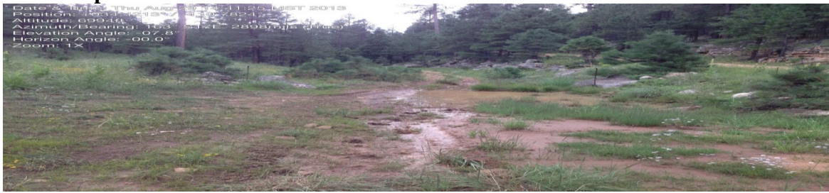
Figure 3 - User created road along stream channel in Little Springs Canyon. The road crosses the channel numerous times before exiting the valley bottom via system roads 1.1 miles upstream.
