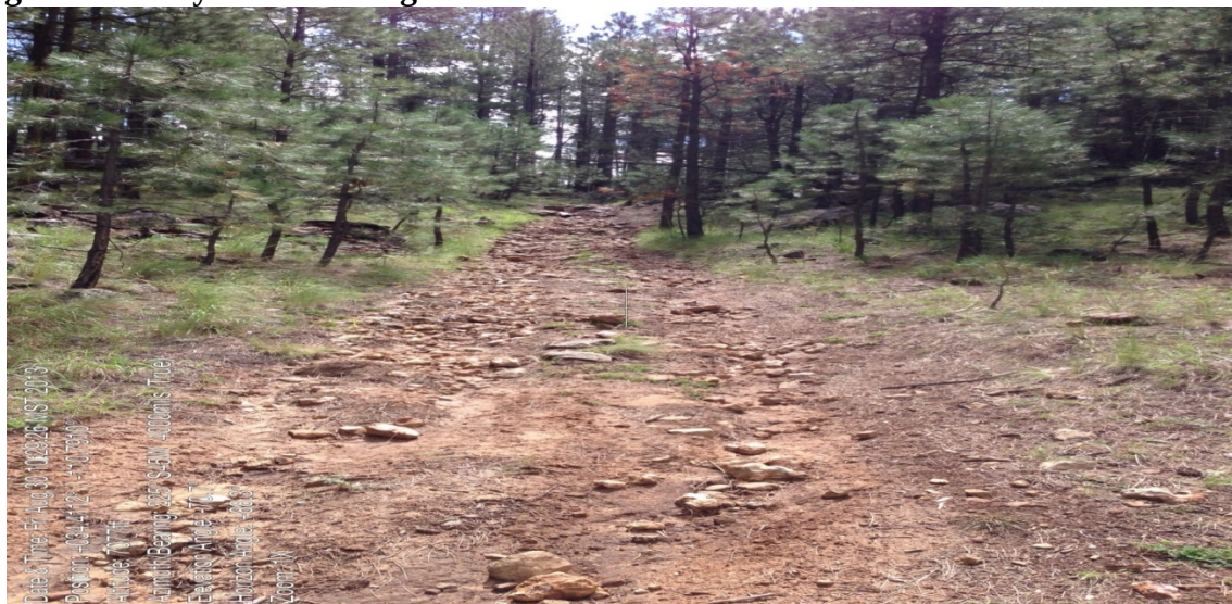
Figure 2 - Gully erosion along FR9527
