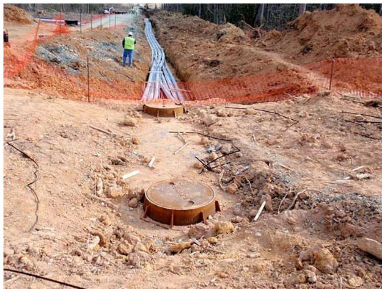
Figure 2.4-2. Example of trenching for underground electric transmission line installation without trench boxes (Dominion)
