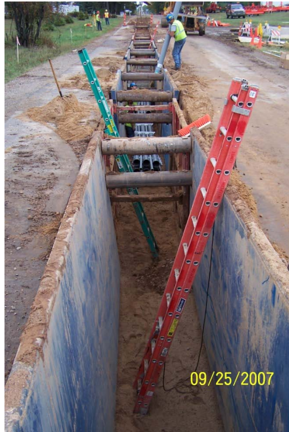
Figure 2.4-1. Example of trenching for underground electric transmission line installation using trench boxes (ATC photo).
