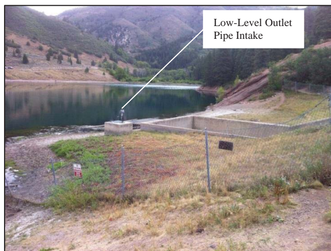
Figure 1-4. Low-Level Outlet Pipe Intake
