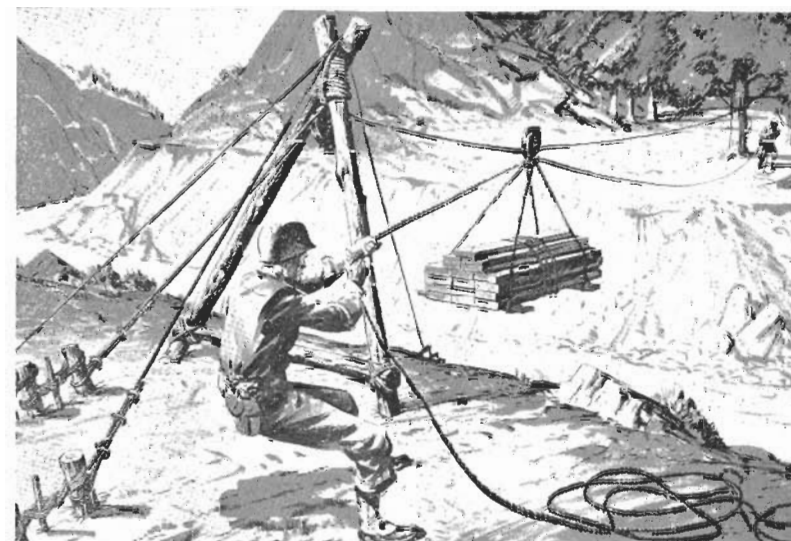
FIGURE 5. Erection cableway. This is used to transport material to the far side and to transfer personnel during erection.
