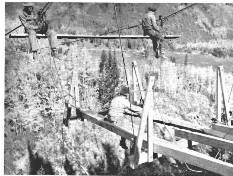
FIGURE 30. Placing stringers. Stringers must be placed from temporary scaffold plank. After the stringers are placed and nailed into position, the erection-scaffold party receives next hanger assembly and goes forward to next panel point.
