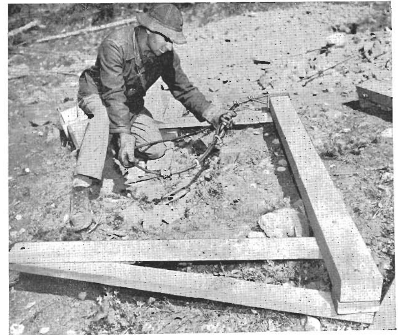
FIGURE 26. Assembled hanger. Hanger is assembled on near side and given to far side party to be installed.
