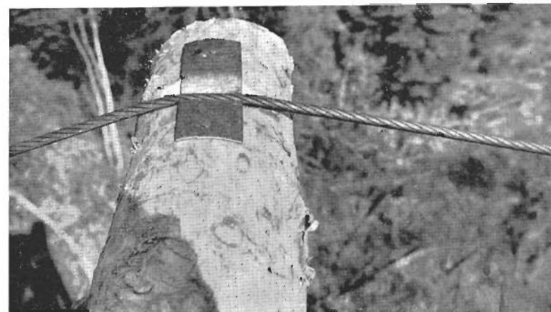
FIGURE 8. Saddle strap for improvised tower type-2. Used to position and steady main cable on tower cap and to prevent the cable from shearing or wearing into the log.
