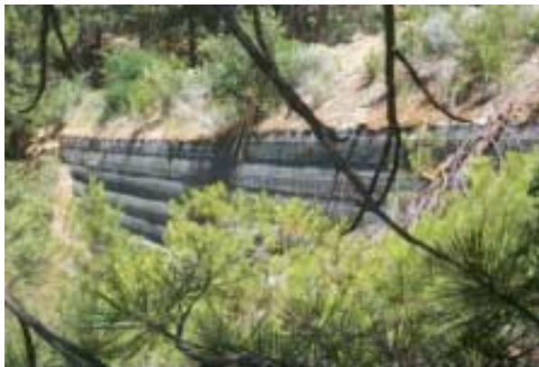
Figure 11—Retaining wall at the Sierra National Forest site.
