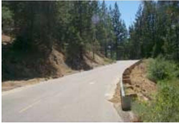
Figure 10—Sierra National Forest site. The drain is installed along the inside edge of the road.
