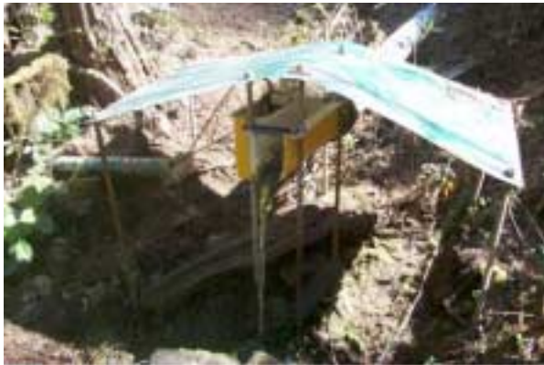
Figure 7—Flume at drain outlet. The water level in the stilling basin on the left side of the flume is measured and converted to a flow volume.
