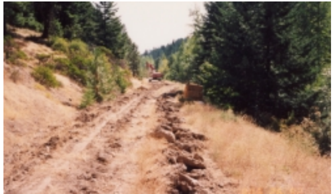
Figure 1—The berm blocking the road was removed to allow fertilizer and bales of mulching straw to be placed every tenth of a mile.
