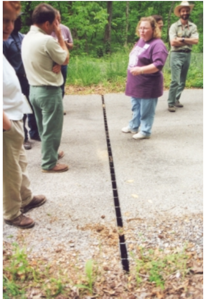
Figure 22—Closeup view of the slot in the roadbed.
