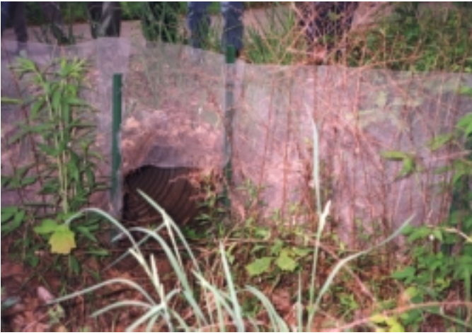
Figure 23—A culvert was installed under the road with plastic webbing to guide the reptiles into the culvert.
