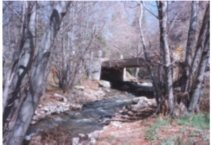
Figure 12—Four precast, 40-ft concrete, single-lane bridges were constructed to replace the natural water crossings and improve aquatic life.
