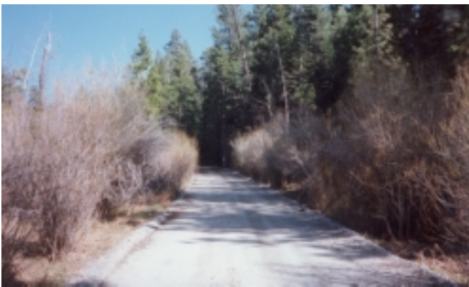
Figure 15—The roadbed was rebuilt using nonwoven geotextile, coarse drain rock, and 3/4-in surfacing aggregate to make a dry road surface.
