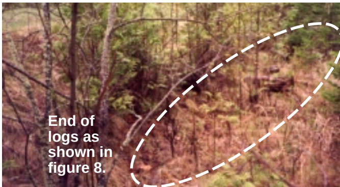
Figure 9—Log corduroy (selected area) was used for cross drainage on this road.
