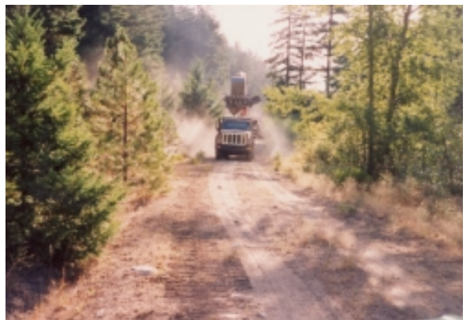
Figure 2—The excavator pulled culverts from the front (junction) of the road to the back.
