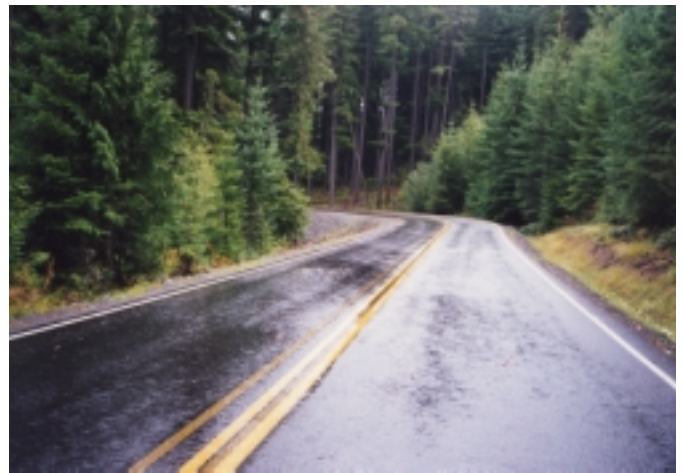
Figure 17—The newly relocated Greenwater River Road.
