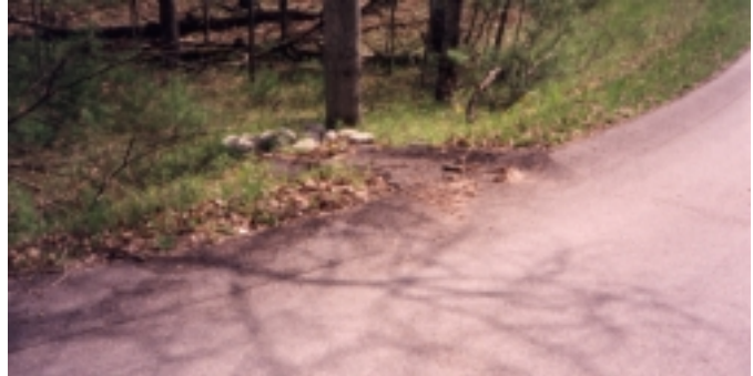
Figure 6—Curbing and drainage structures channel runoff flows off the roadway and into fields or sediment beds.
