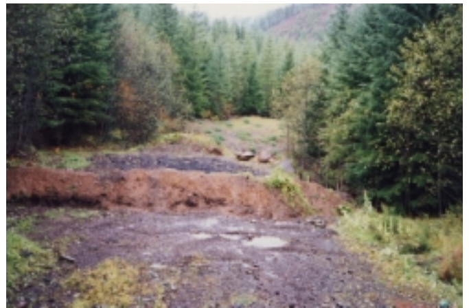
Figure 18—By blocking the two entrances, pulling all culverts, and seeding and mulching the roadbed and sideslopes, the upper road closure affected only 2.9 mi of the existing road.
