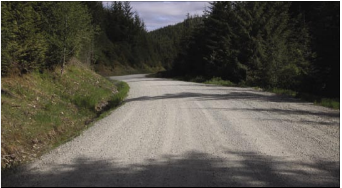
Figure 6—Maintenance level 4 road with double lanes, gravel surface, and gravel shoulders.
