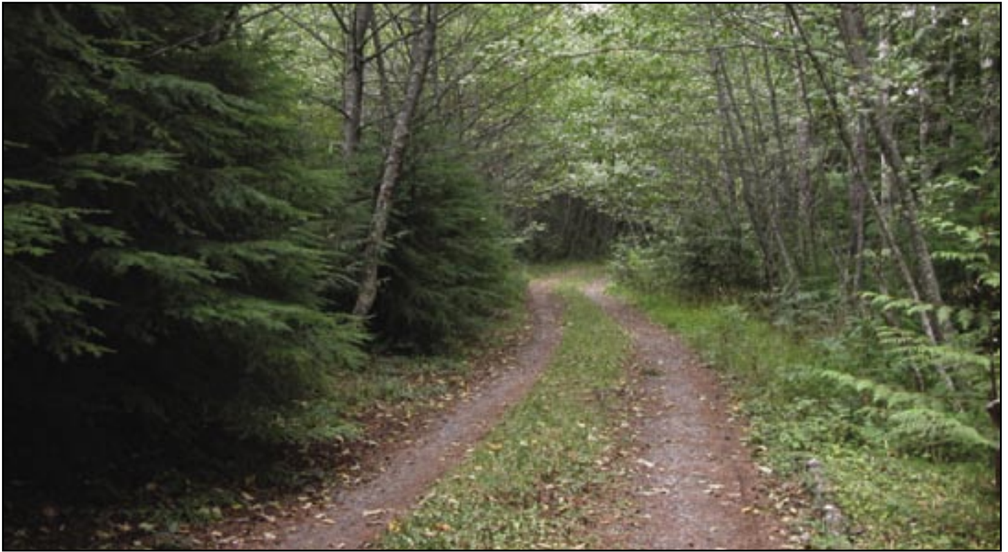
Figure 20—Maintenance level 3 road with single lane, gravel surface, and no shoulders.
