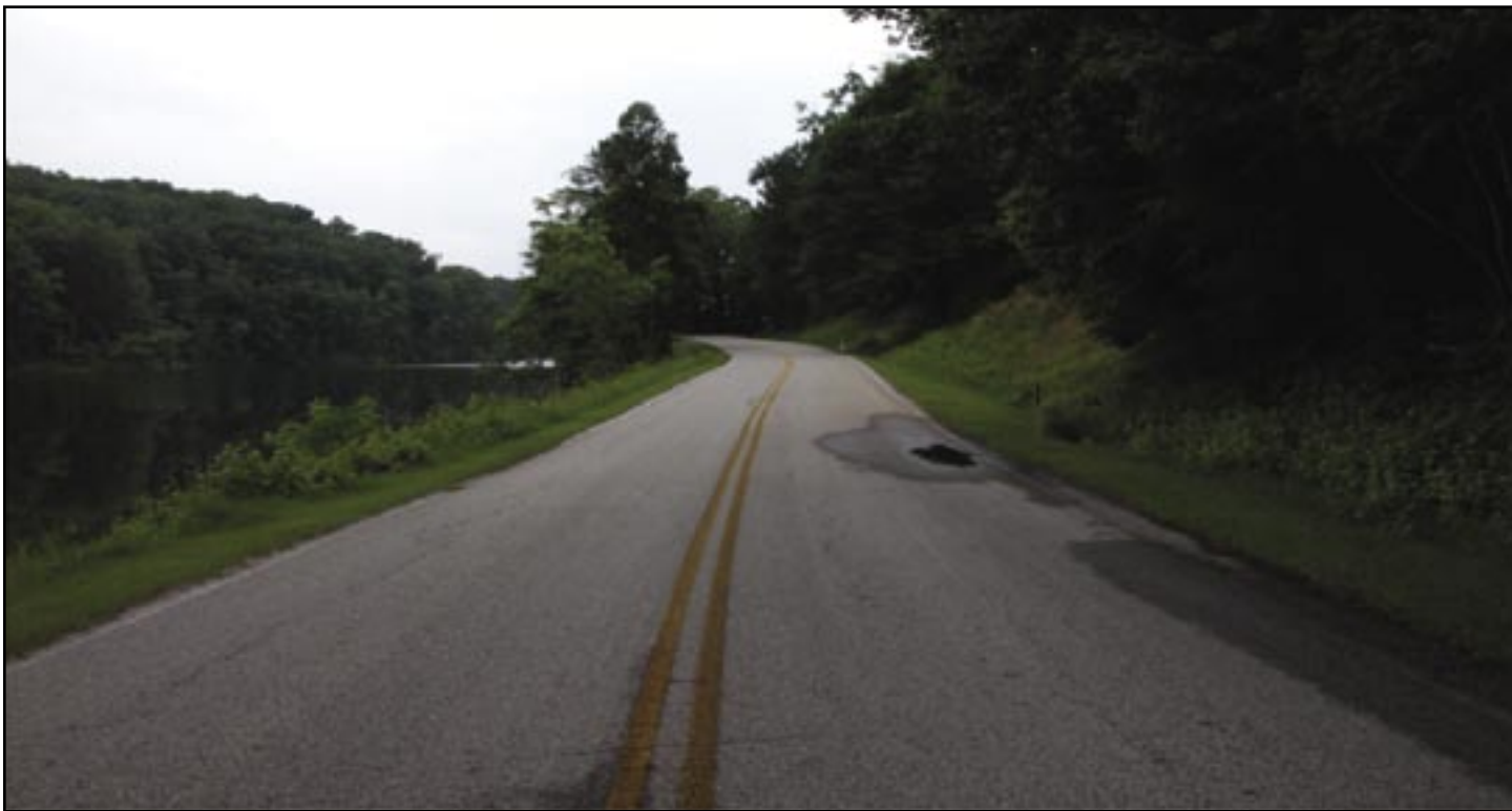
Figure 2—Maintenance level 5 road with double lanes, asphalt surface, and unpaved shoulders.
