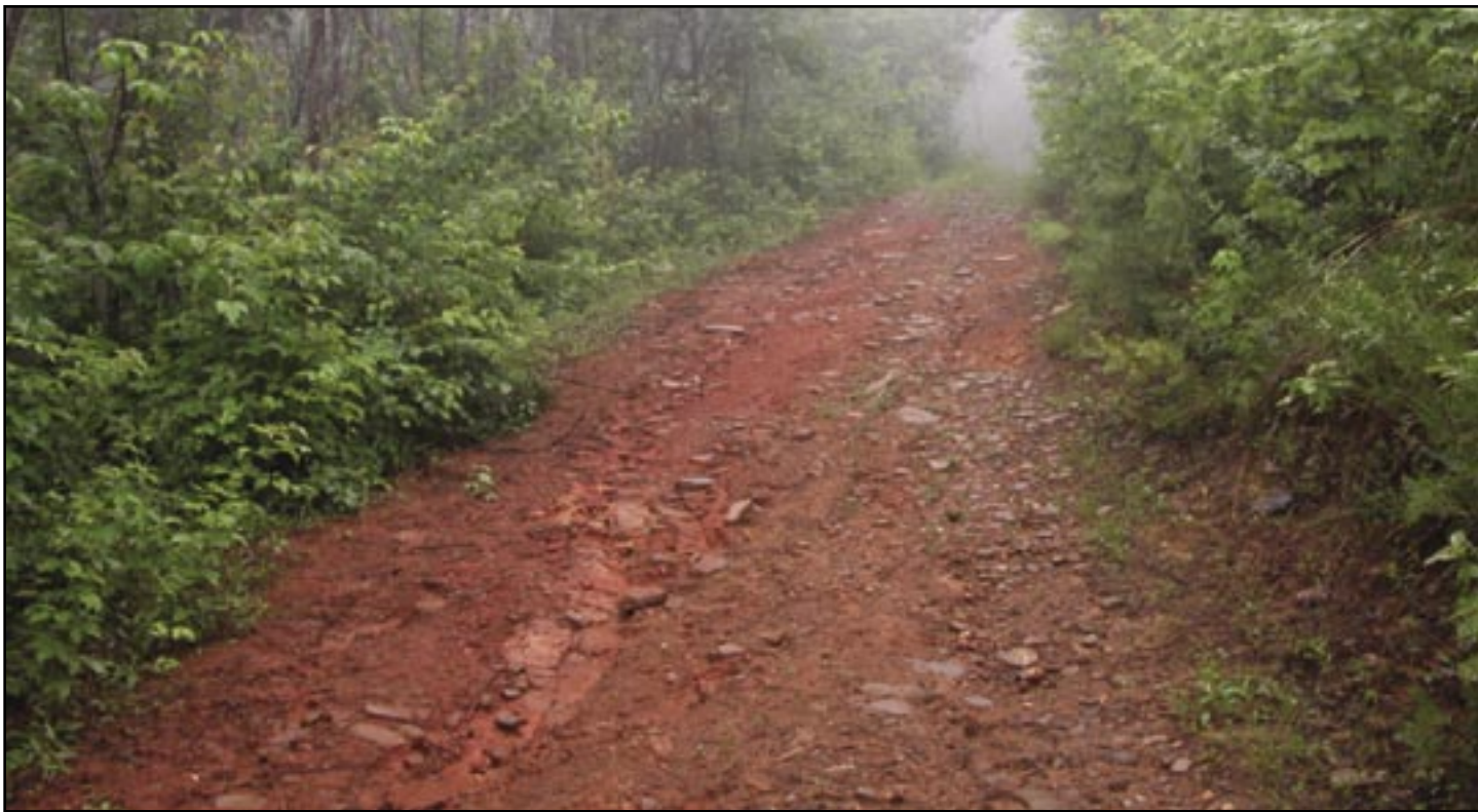
Figure 22—Maintenance level 2 road with single lane, pit-run surface, no shoulders.
