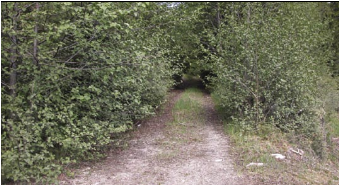
Figure 24—Maintenance level 2 road with single lane, pit-run surface, no shoulders, and suitable for high-clearance vehicles, but with very limited sight distance due to extreme vegetative encroachment.
