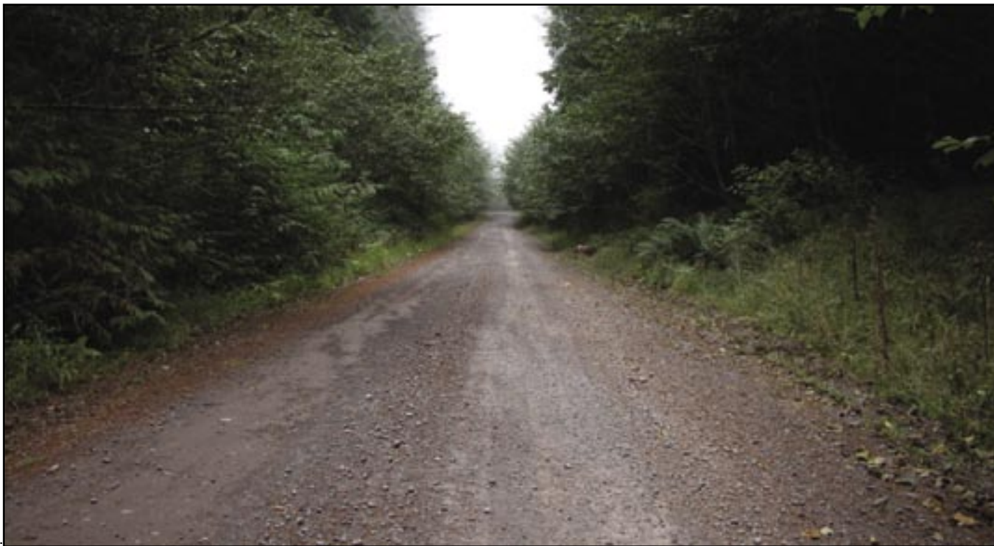
Figure 15—Maintenance level 3 road with single lane, gravel surface, and gravel shoulders.
