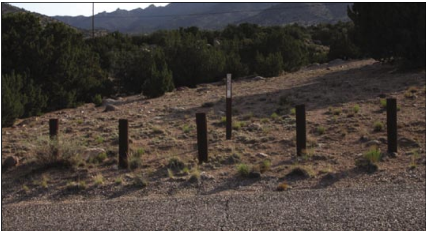
Figure 31—Maintenance level 1 road that has been blocked to highway vehicle traffic by posts. Also includes a sign prohibiting motorized vehicles.
