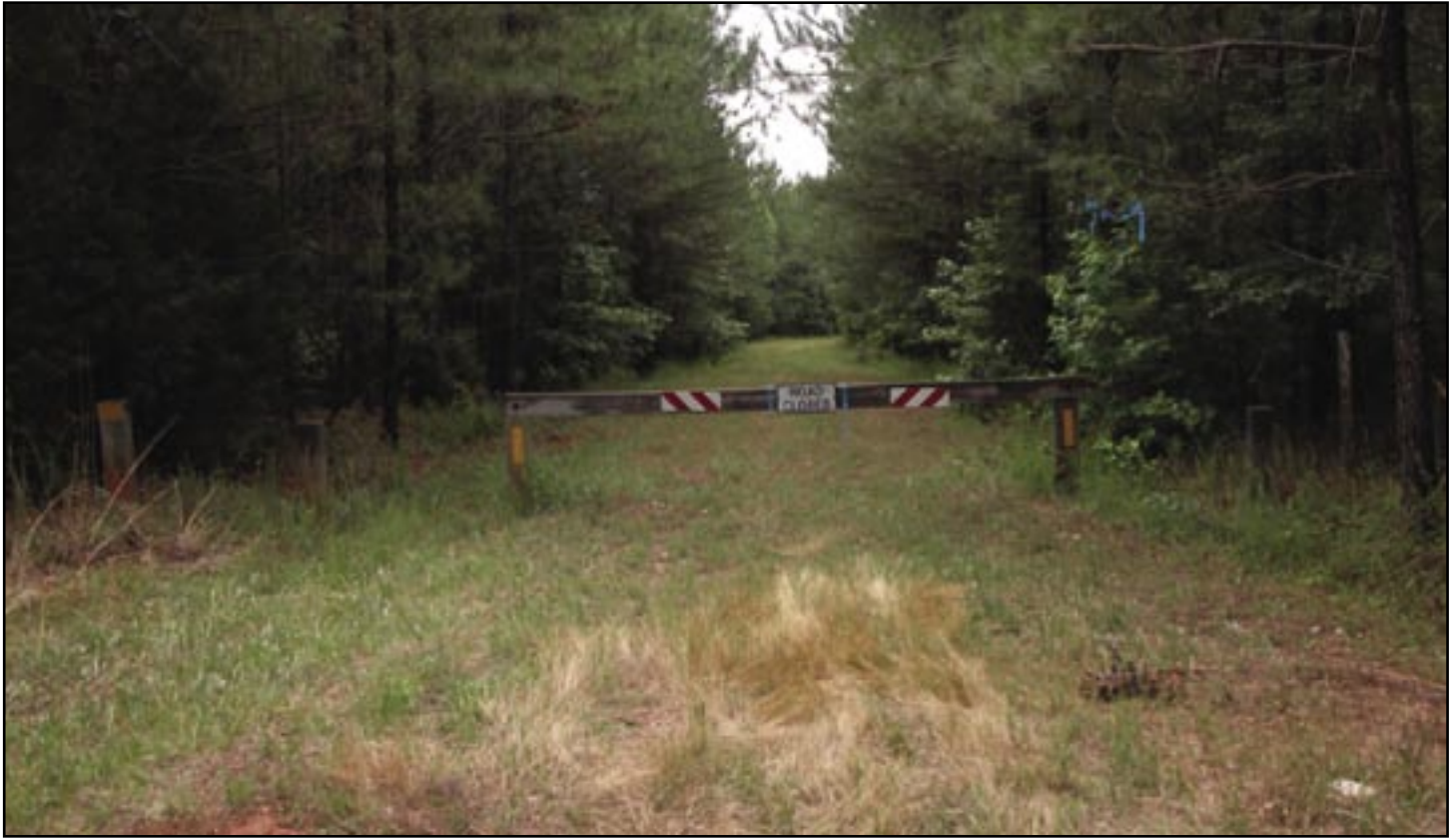
Figure 34—Maintenance level 1 road with highway vehicle traffic eliminated by a barricade and posts.
