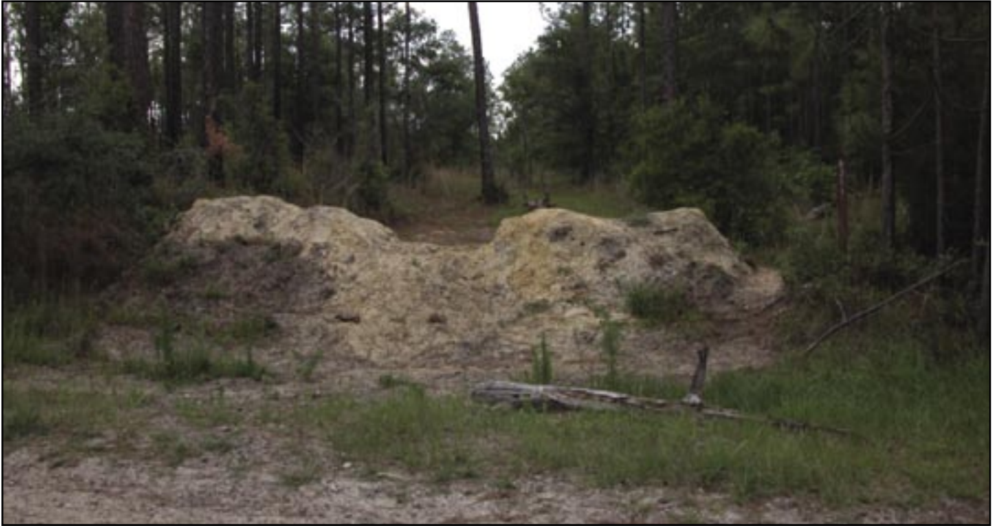
Figure 29—Maintenance level 1 road that has been blocked to highway vehicle traffic by an earth mound.
