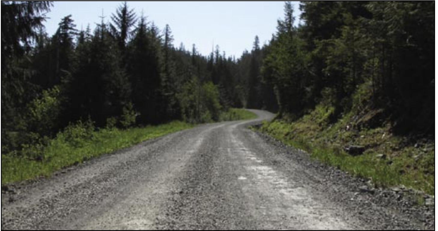
Figure 13—Maintenance level 3 road with single lane, gravel surface, and gravel shoulders.
