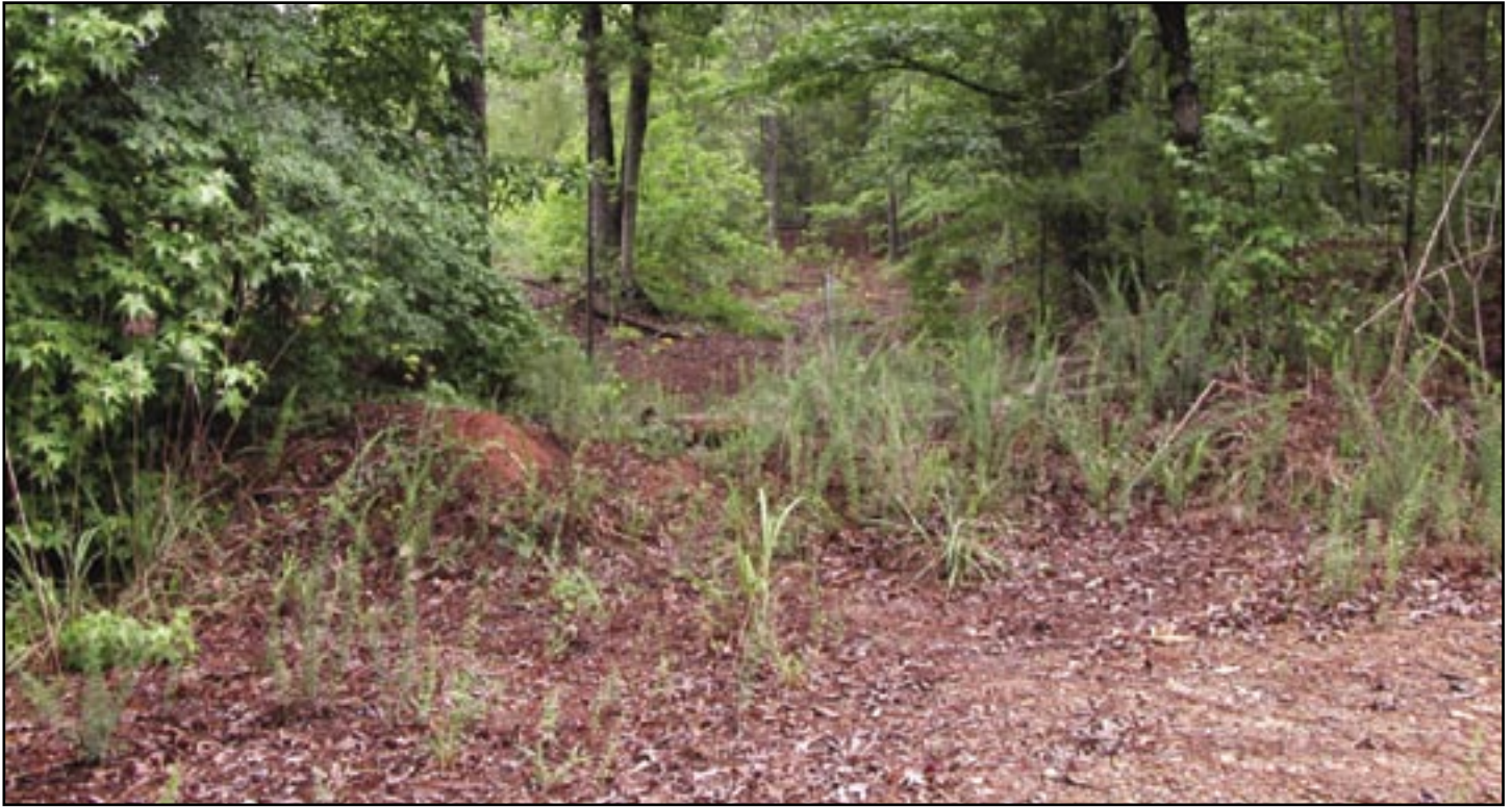
Figure 33—Maintenance level 1 road with the highway vehicle traffic eliminated by a vegetated earth mound, which both disguises and physically blocks the road.
