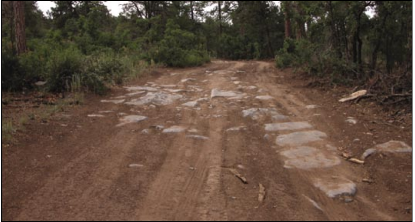
Figure 25—Maintenance level 2 road with single lane, native surface, no shoulders, and suitable for high-clearance vehicles only.
