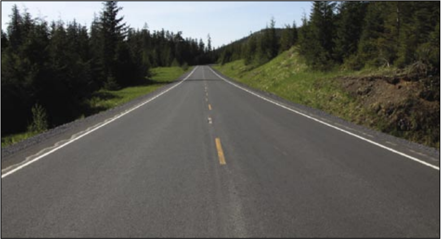
Figure 1—Maintenance level 5 road with double lanes, hot-mix asphalt surface, and asphalt- and rock-stabilized shoulders.
