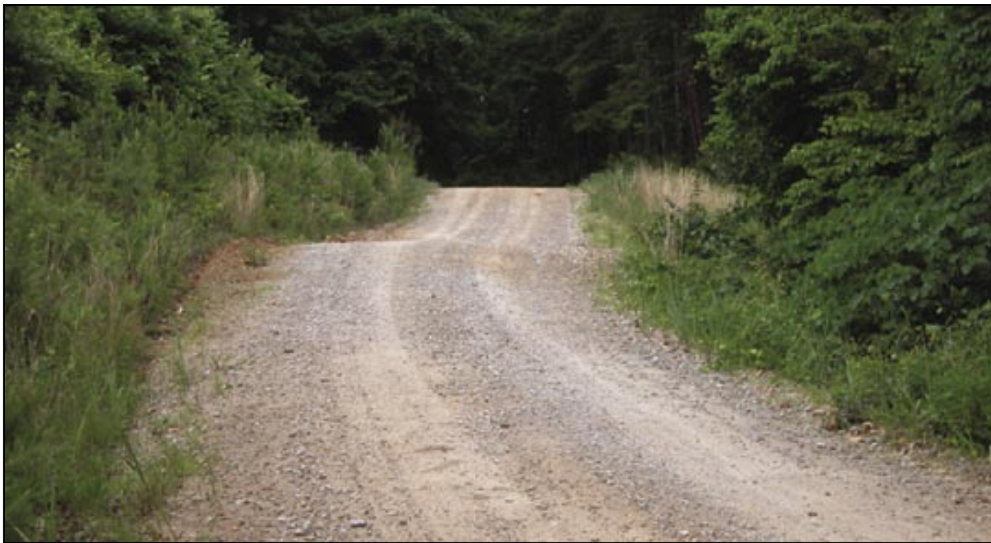
Figure 16—Maintenance level 3 road with single lane, gravel surface, no shoulders, and a cross drain dip.
