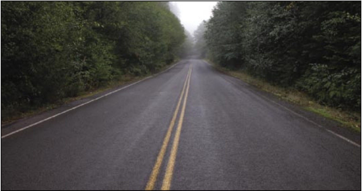
Figure 5—Maintenance level 5 road with double lanes, asphalt surface, and asphalt shoulders.
