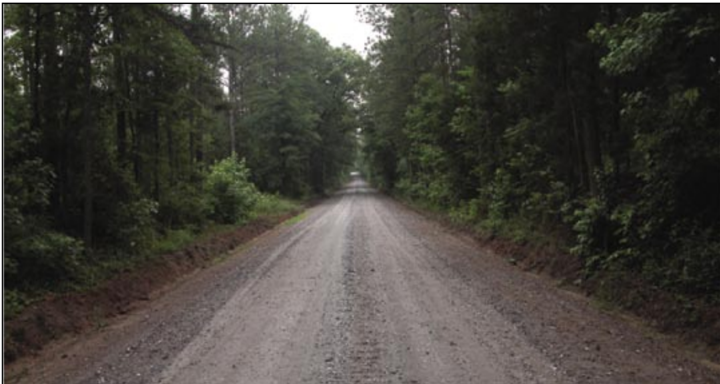
Figure 11—Maintenance level 4 road with single lane, gravel surface, and gravel shoulders.
