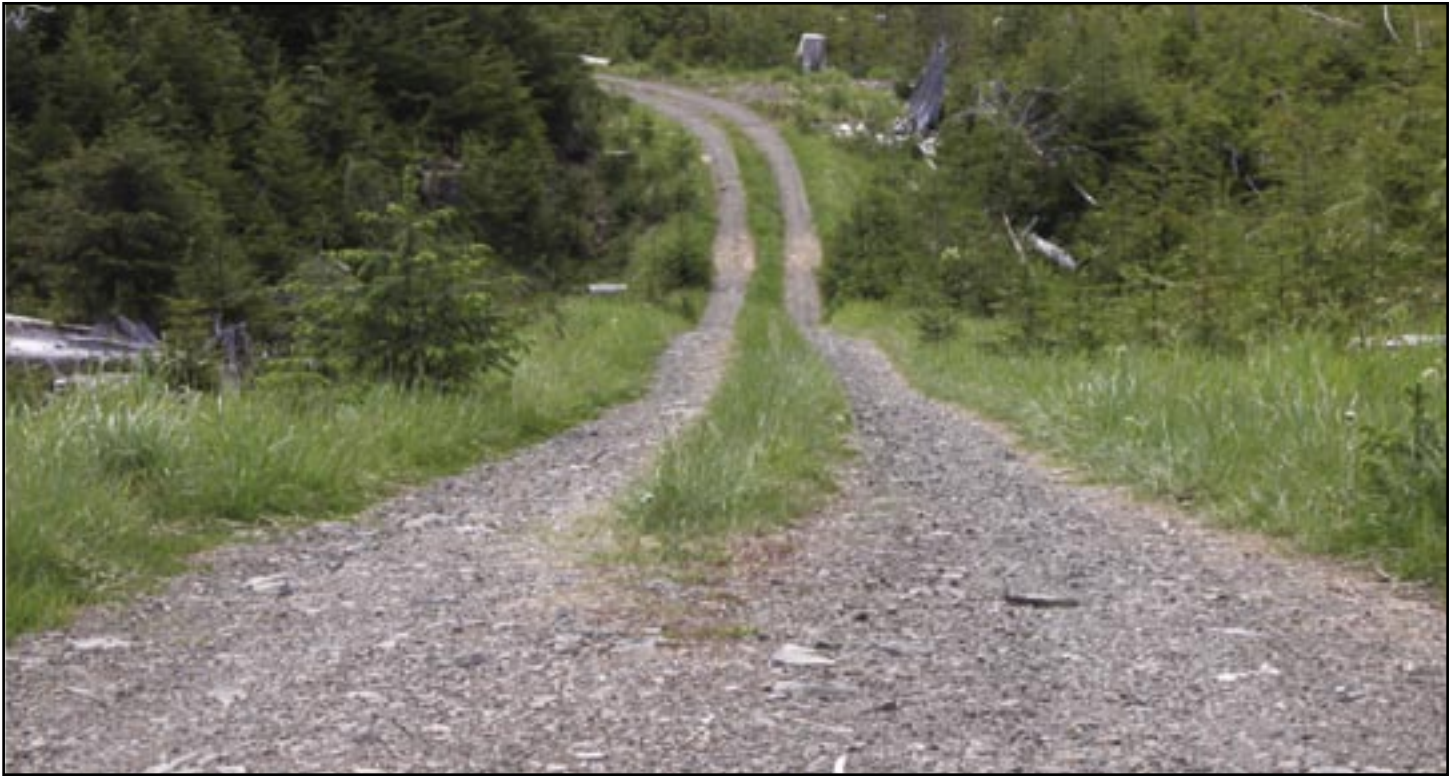
Figure 19—Maintenance level 3 road with single lane, gravel surface, and no shoulders.
