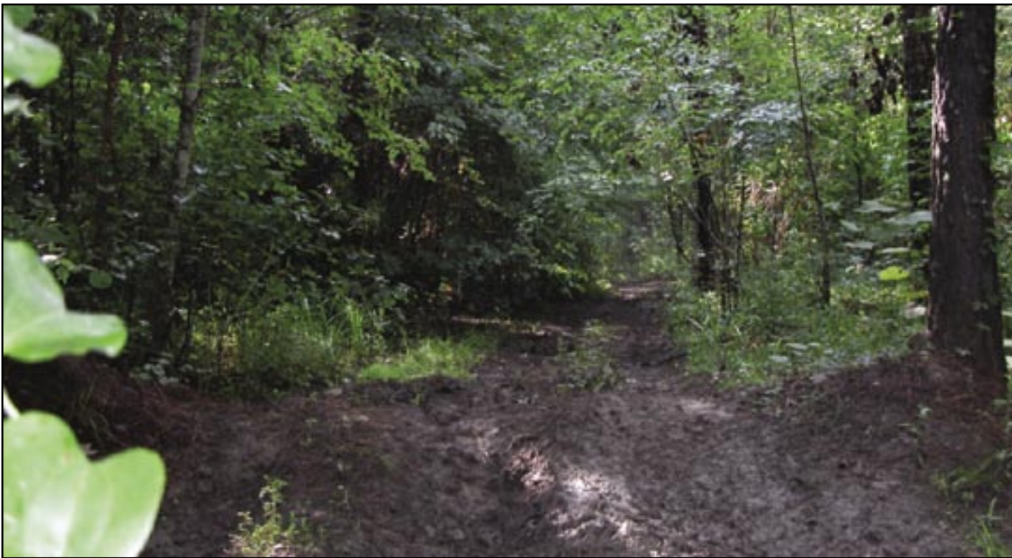
Figure 26—Maintenance level 2 road with single lane, native surface, no shoulders, and suitable for high-clearance vehicles only.
