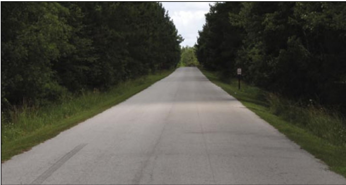
Figure 3—Maintenance level 5 road with double lanes, chip-seal surface, and unpaved shoulders.
