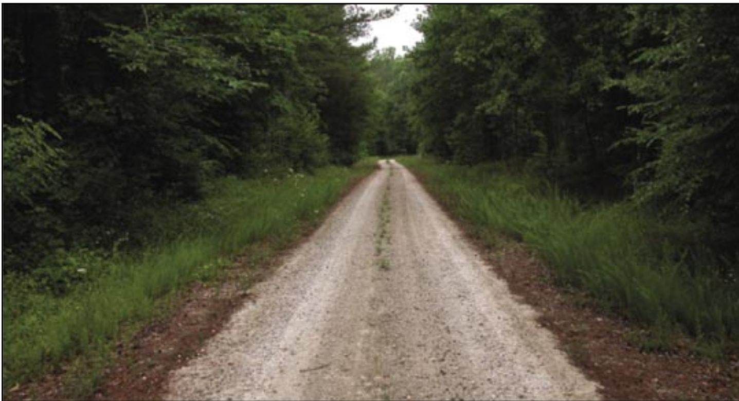
Figure 17—Maintenance level 3 road with single lane, gravel surface, and no shoulders.
