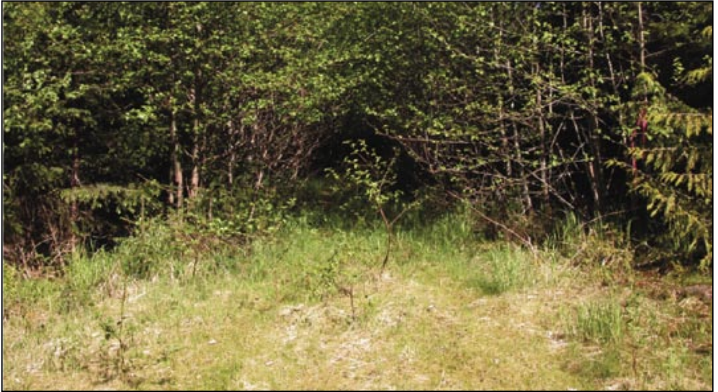
Figure 32—Maintenance level 1 road that has been blocked to highway vehicle traffic by natural vegetative overgrowth.
