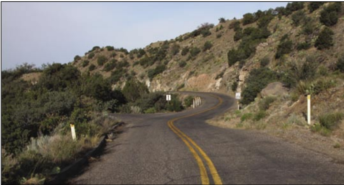
Figure 7—Maintenance level 4 road with double lanes, asphalt surface, and no shoulders.
