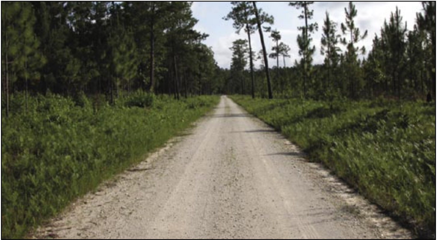
Figure 12—Maintenance level 3 road with single lane, gravel surface, and gravel shoulders.
