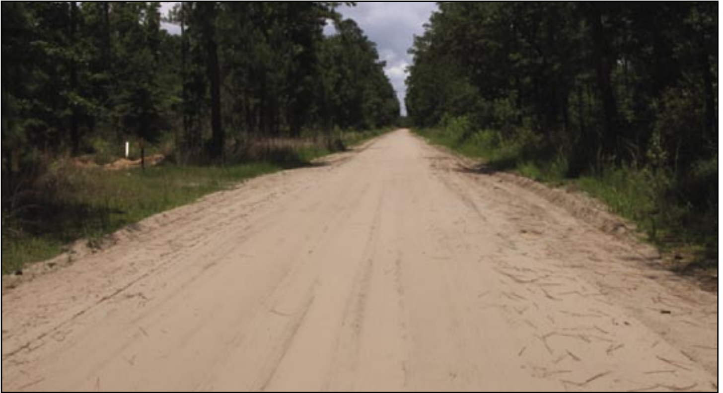
Figure 18—Maintenance level 3 road with double lanes and native road surface with shoulders.
