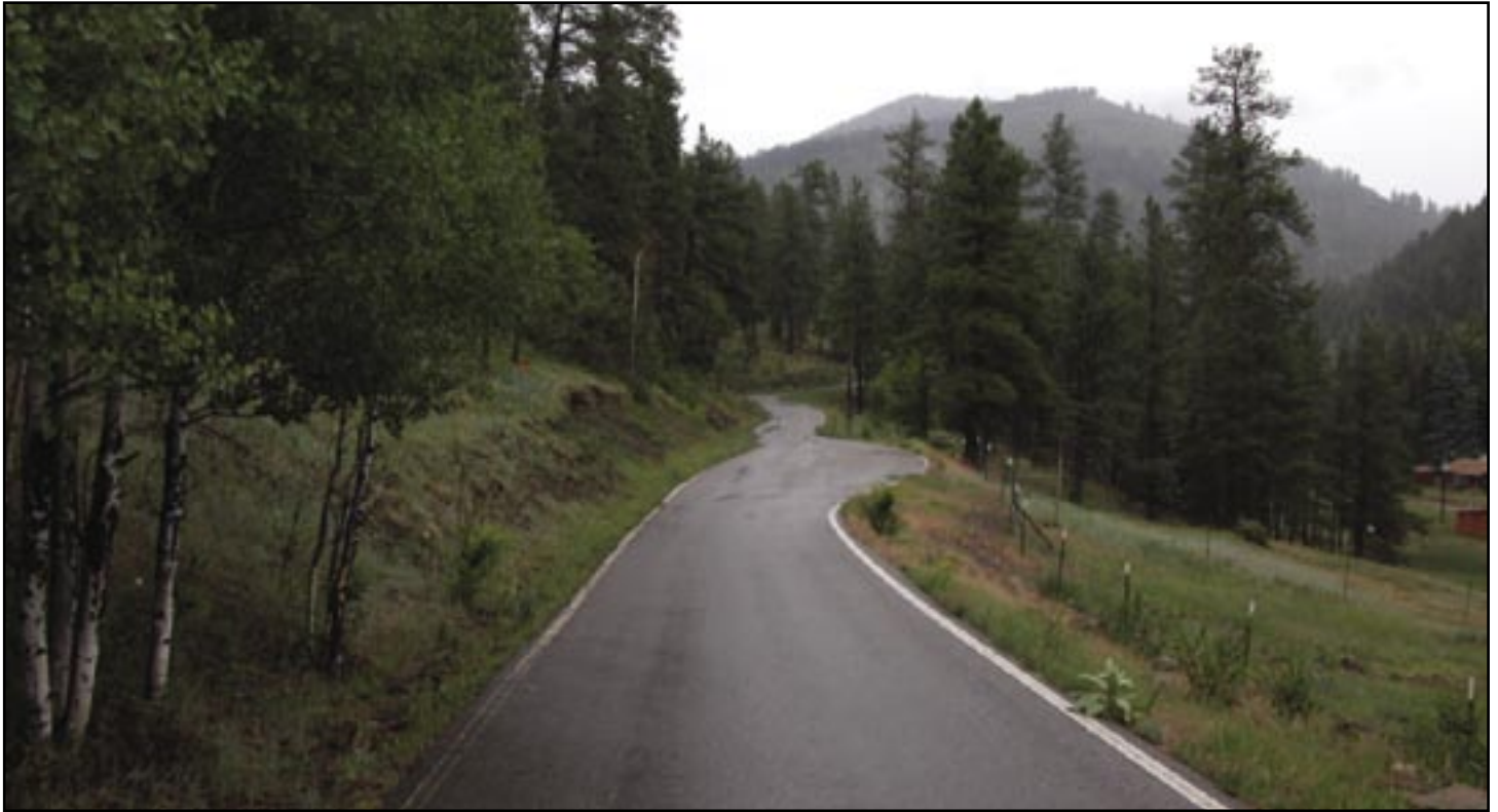
Figure 8—Maintenance level 4 road with a single lane, asphalt surface, no shoulders, and paved turnouts.
