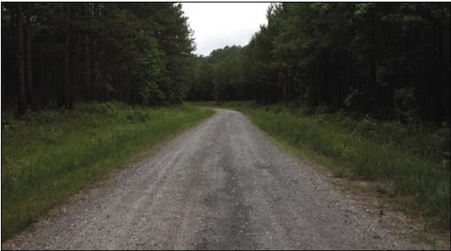
Figure 14—Maintenance level 3 road with single lane, gravel surface, and gravel shoulders.
