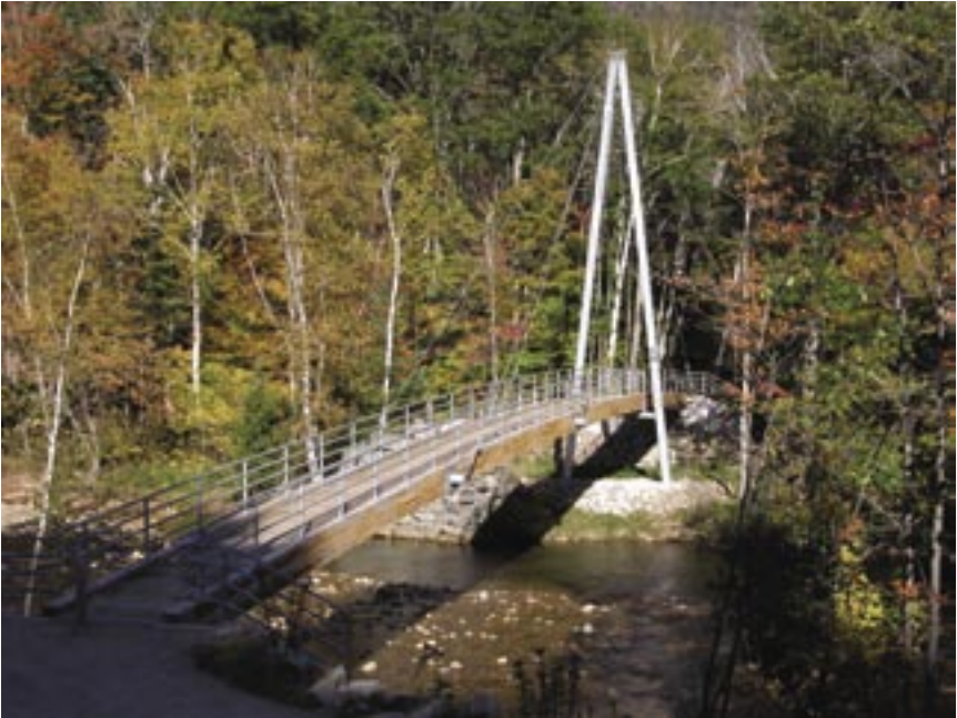
Asymmetric bridge, White Mountain National Forest.
