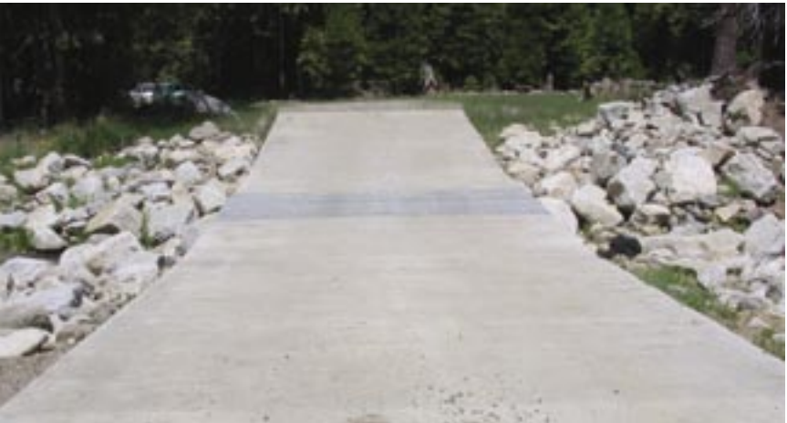
Vented-ford crossing with removable steel deck.
