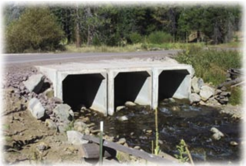
Precast triple-box culvert.
