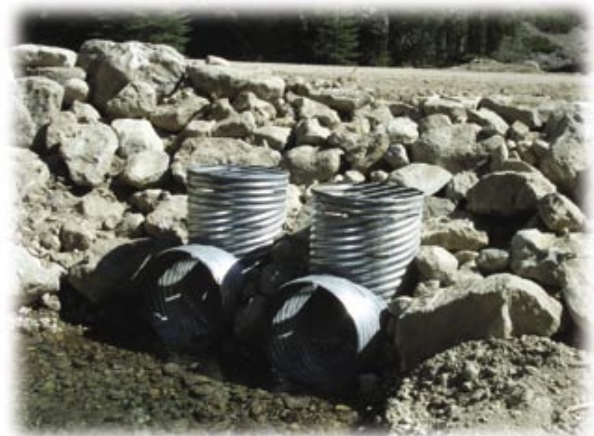
Modification of existing culverts to prevent plugging.
