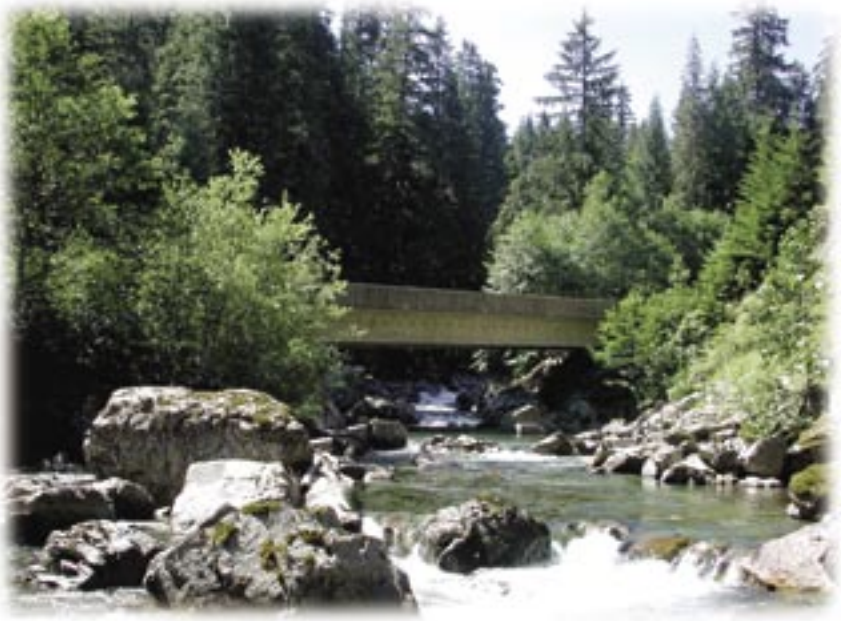
Single-span concrete-girder bridge.
