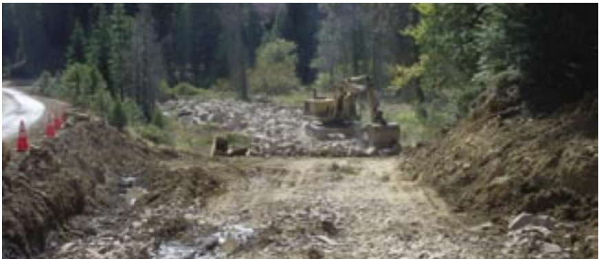
Permeable fill during construction.
