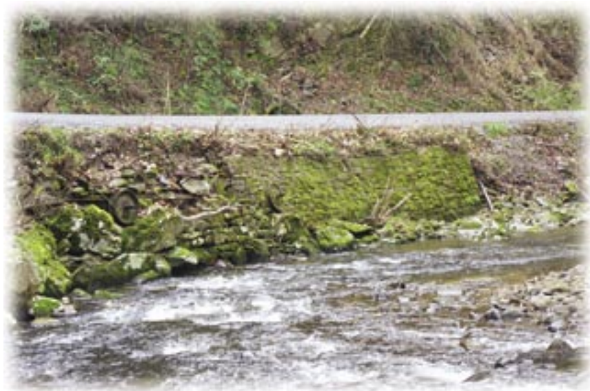
Rock retaining wall.
