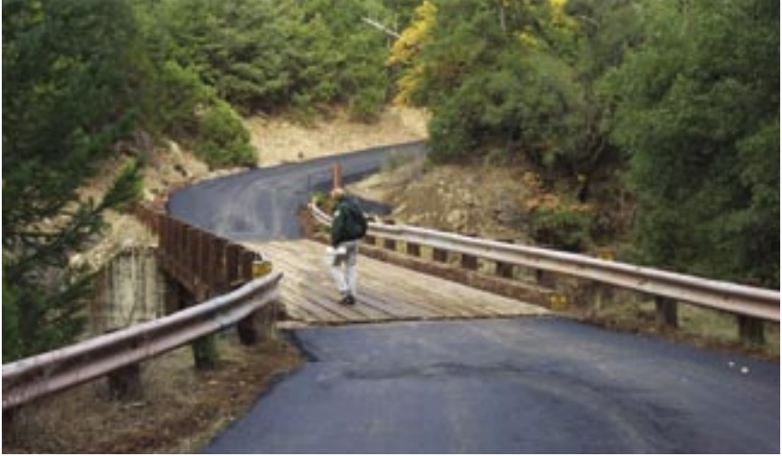
Paved bridge approach.
