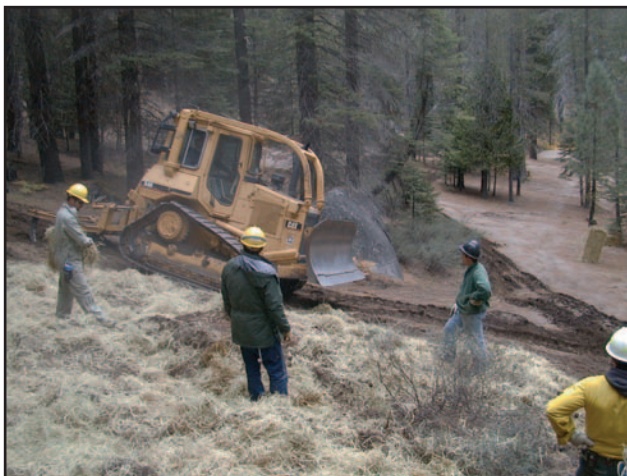
Figure 16—Big Silver and Bassi Creeks watershed restoration project repaired damage done by uncontrolled OHV use. Families have begun to return to the area to picnic and hike to Bassi Falls.
