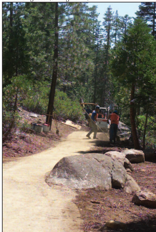
Figure 27—SMUD contracted and oversaw construction of this accessible trail.
