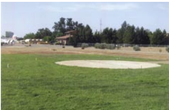
Figure 33—Example of a well-turfed heliport.
