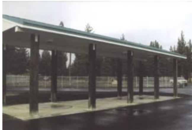
Figure 25—Retardant storage structure.
