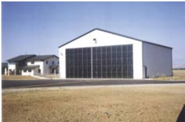
Figure 26—Hangar (Porterville, CA).
