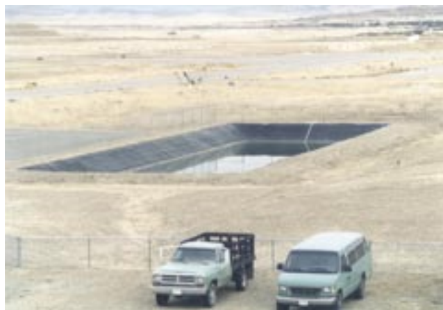
Figure 75—Evaporation lagoon.
