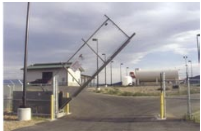
Figure 76—Base fencing and security gate (Helena, MT).
