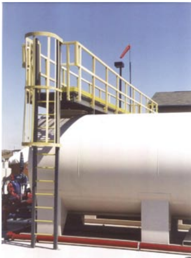
Figure 36—Platform over tanks (JEFFCO, CO).
