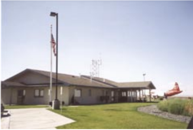
Figure 67—Retardant base operations office (Moses Lake, WA).
