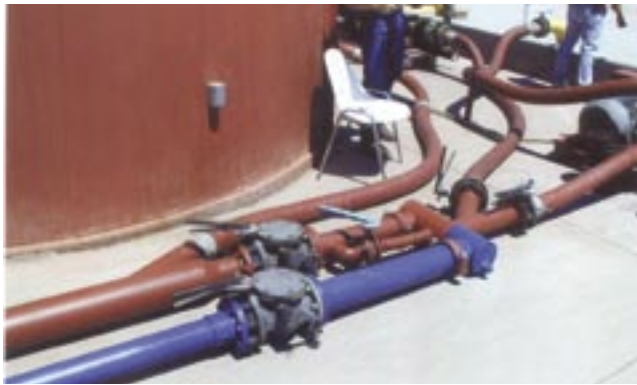
Figure 44—Inline proportioner, orifice blender (Redmond, OR).
