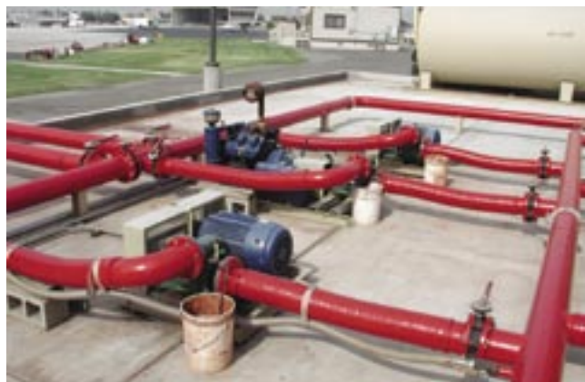
Figure 48—Electric- and gasoline-powered retardant pumps with vibration isolating flexible hose (San Bernardino, CA).
