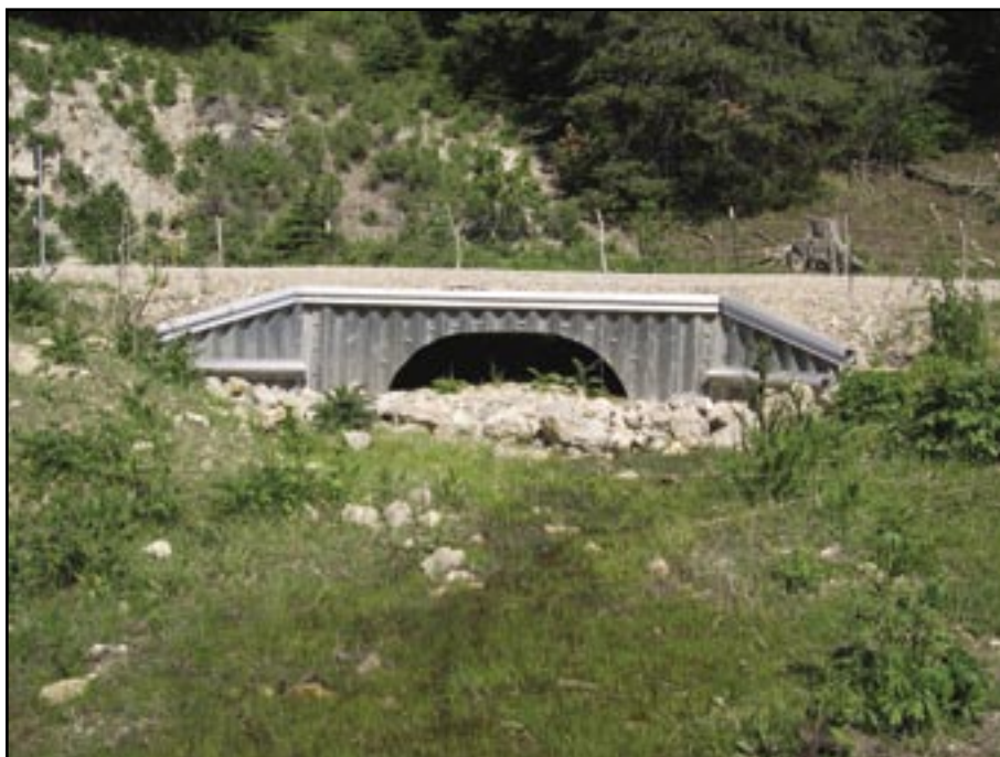
Figure 6—Aluminum pipe arch outlet. Photo taken June 2005. Note large arch opening requires only infrequent maintenance despite relatively large springflows. We constructed the road prism of 2- to 3-foot-deep permeable rock fill. The listed plant, Sacramento Mountain thistle ( Cirsium vinaceum ) is in the outlet of the structure.
