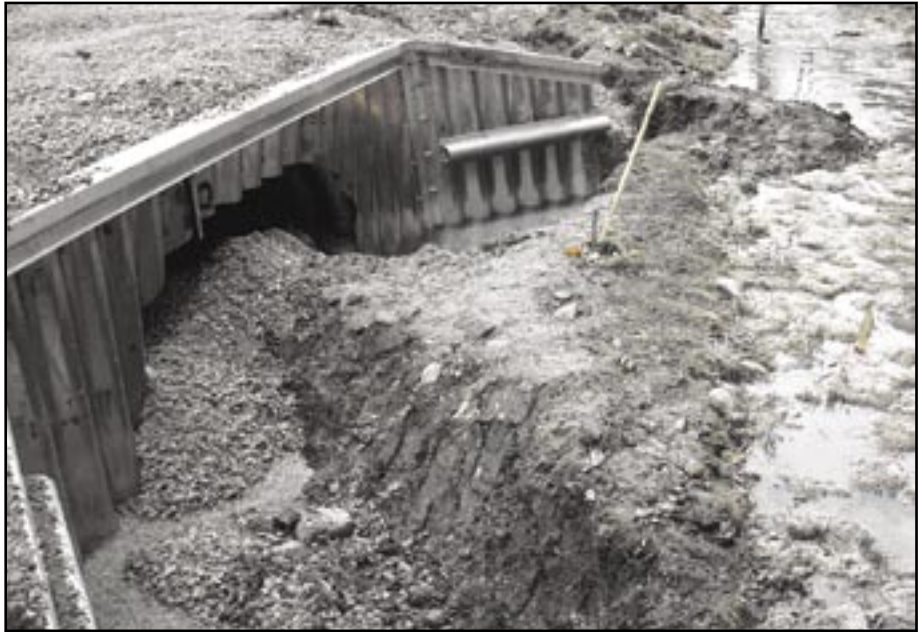
Figure 4—Aluminum pipe arch inlet during construction. Note that springwater is still diverted down the ditch to minimize flow through disturbed area. We did not allow the contractor to divert water with equipment. USDA Forest Service personnel diverted the water by hand by to minimize disturbance to the habitat.
