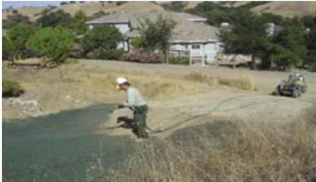
Figure 14—Using the sprayer to hydromulch. Tank is barely visible behind the ATV.
