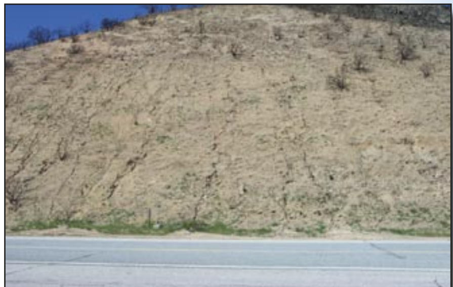
Figure 2-8—Rill erosion is prevalent on this cutslope due to lack of soil cover. Steep and long slope lengths without vegetation or soil cover are susceptible to accelerated erosion.
