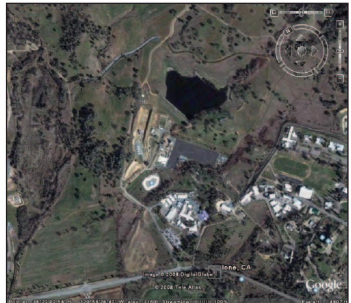
Figure 1—Lone location photo.
