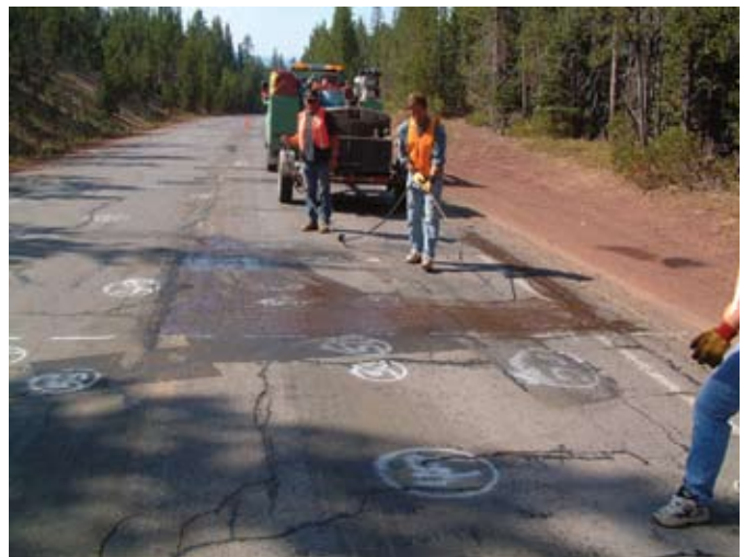
Figure 6—A quick-set tack was applied to GlasGrid test cells to ensure good bond.
