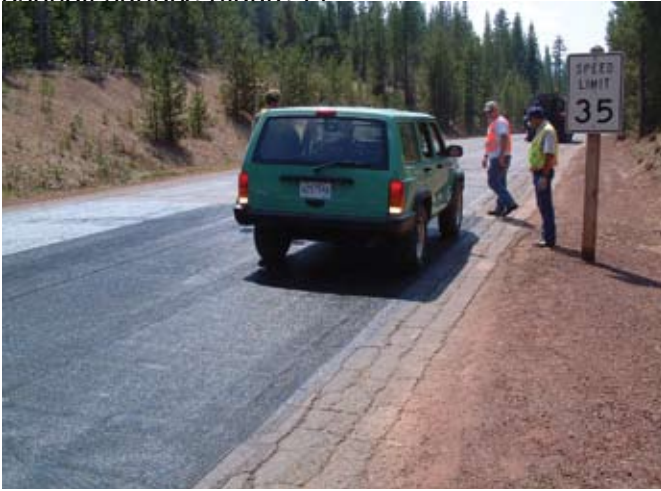
Figure 7—Seating the GlasGrid by rolling with a light-duty vehicle.
