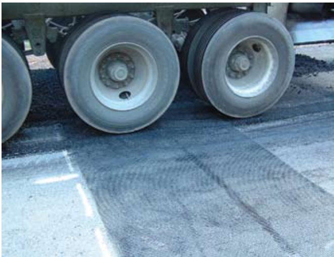
Figure 8—GlasGrid remained bonded to the underlying surface during paving operations.
