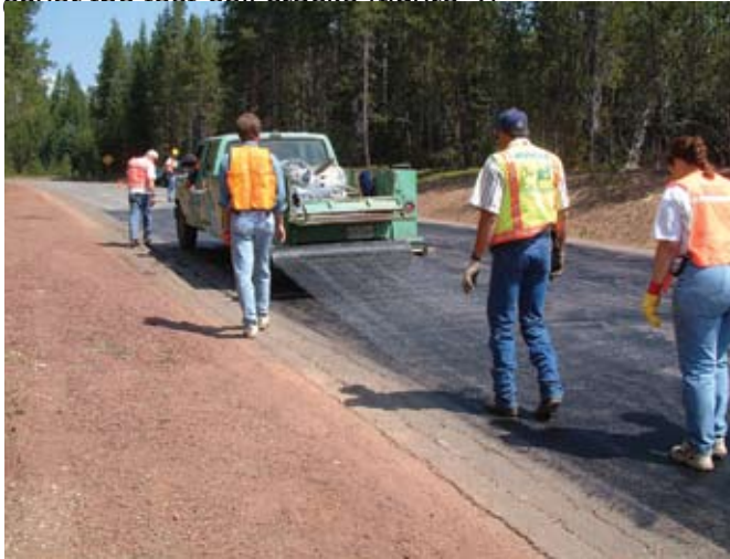
Figure 3—Placing GlasGrid from the spool, which is attached to a trailer hitch.
