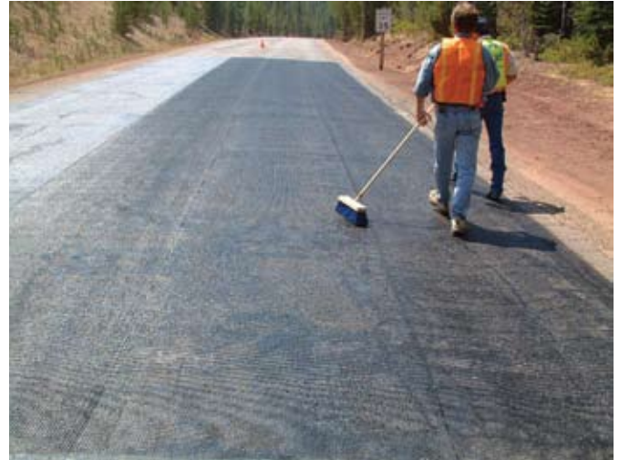
Figure 5—GlasGrid Type 8501 was applied with 100-percent coverage in test section 2. A 2-inch overlap was used at all seams.
