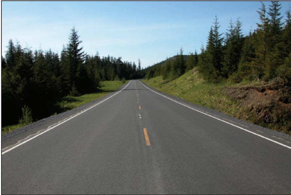
Figure 1—Maintenance level 5 double-lane road with centerlines and edge markings, a hot-mix asphalt surface, and asphalt- and rock-stabilized shoulders. If centerline markings are placed on a road, the no-passing zone markings also shall be placed as determined by an engineering study.
