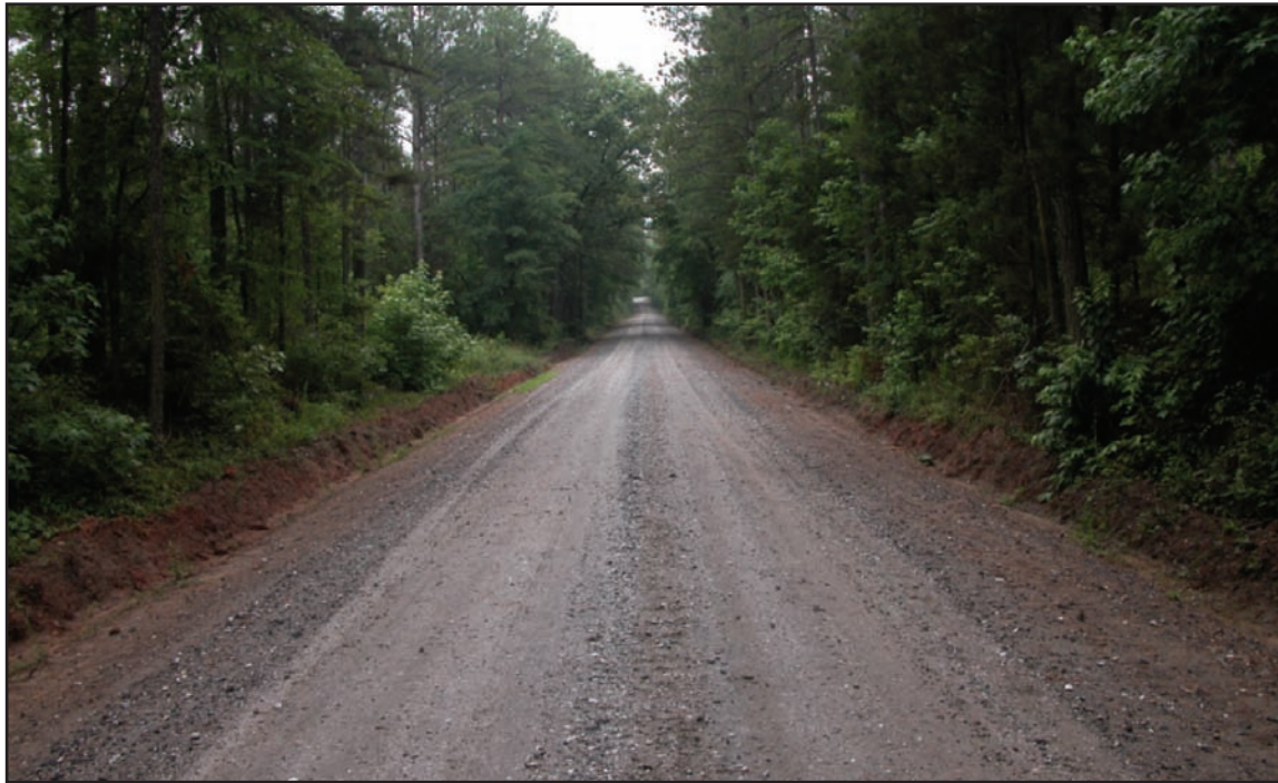
Figure 11—Maintenance level 4 single-lane road with a gravel surface and gravel shoulders with ditches. The ditches have been cleaned out to facilitate proper drainage. Maintain proper crown, repair potholes, and remove washboarding to facilitate drainage and to maintain a moderate degree of user comfort and convenience at moderate travel speeds. Replace surfacing to the depth required for blade maintenance and to prevent wear of the base course. The roadside vegetation is becoming overgrown and should be maintained to provide adequate sight distance.
