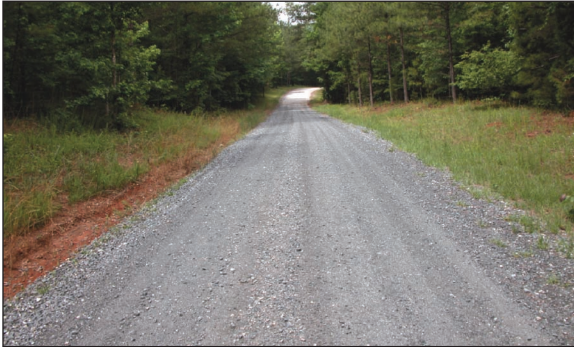
Figure 9—Maintenance level 4 single-lane road with a gravel surface and gravel shoulders. Maintain a proper crown, repair potholes, and remove washboarding to facilitate drainage and to maintain a moderate degree of user comfort and convenience at moderate travel speeds. Maintain ditches to facilitate drainage. The road is free of litter and the maintenance of the roadside vegetation provides adequate sight distance. Curves and other hazards should be marked with warning signs if advised by a documented engineering judgment or engineering study.
