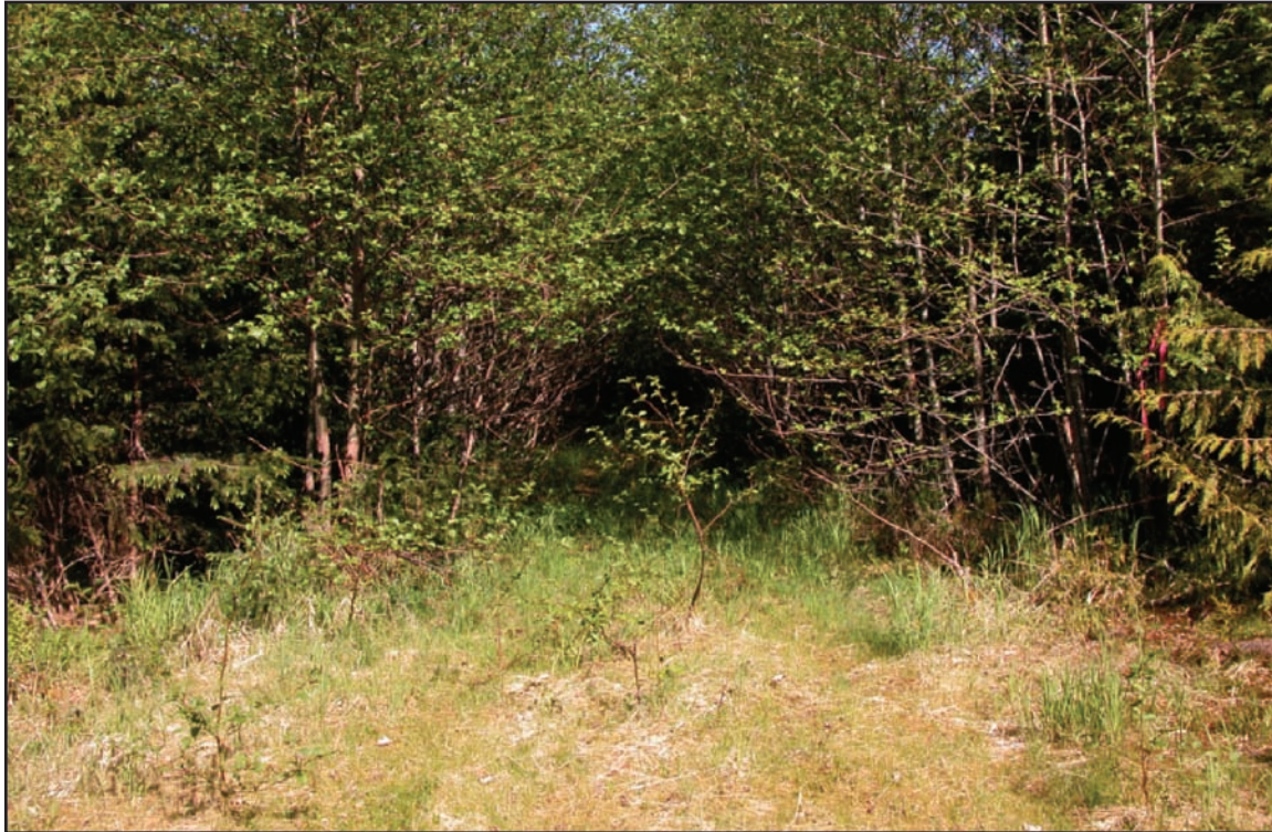
Figure 28—Maintenance level 1 road that has been blocked to motor vehicles by natural vegetative overgrowth. Camouflage is a good alternative when there is limited availability of large rocks or down trees to use as a barrier. Vegetation treatment, such as planting, may be an effective solution in regions with suitable growing conditions.
