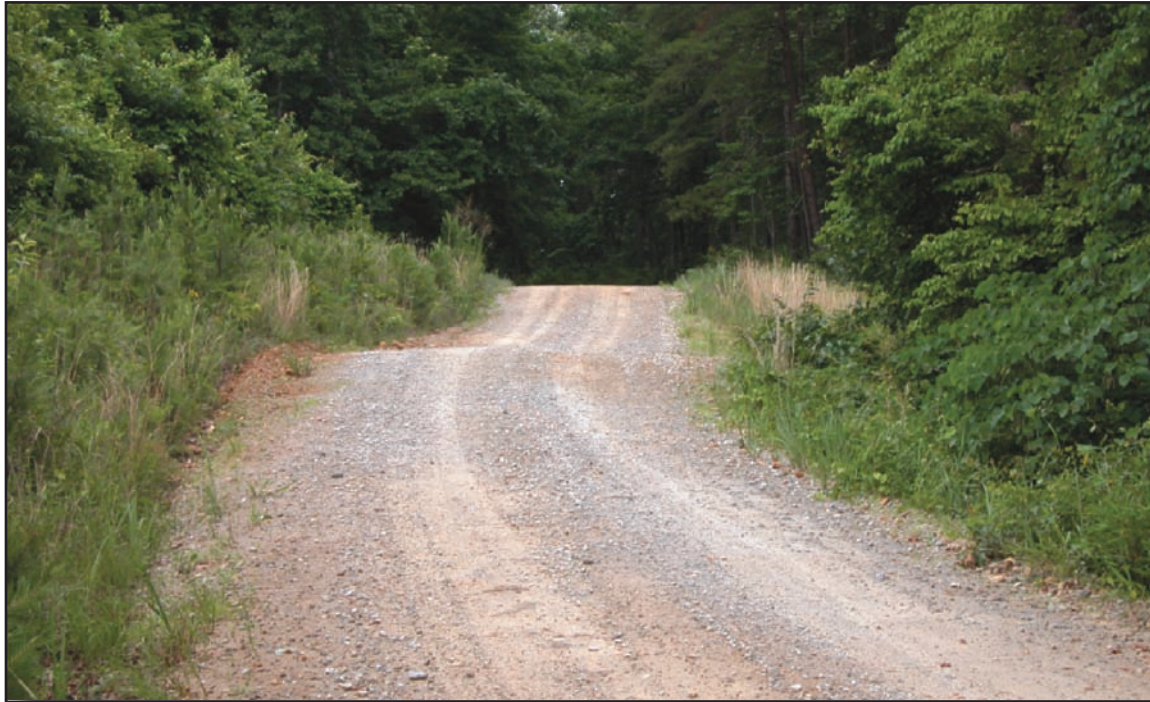
Figure 15—Maintenance level 3 single-lane road with a gravel surface, no shoulders, and a cross-drain dip. Drainage facilities, such as drain dips, should be maintained so they are functional to prevent unacceptable environmental and resource damage and to provide travel by prudent drivers in standard passenger cars. Surface roughness is acceptable if travel by prudent drivers in standard passenger cars is provided. Curves and other hazards should be marked with warning signs if advised by a documented engineering judgment or engineering study.
