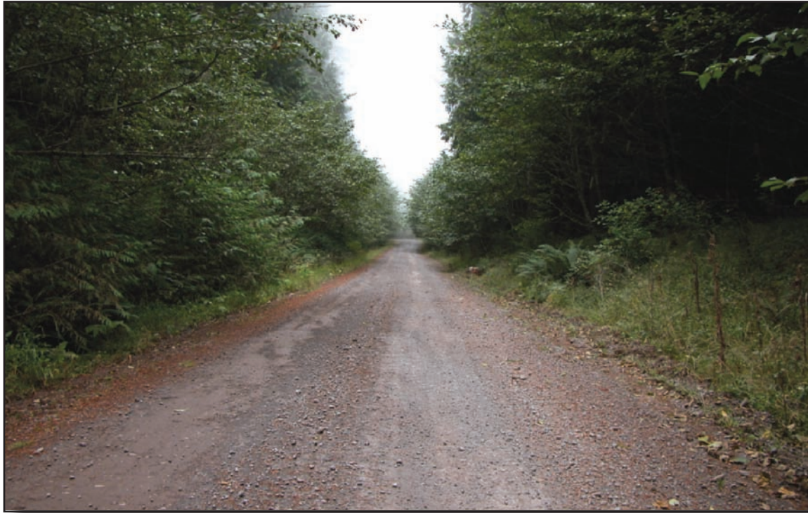
Figure 14—Maintenance level 3 single-lane road with a gravel surface and gravel shoulders. Surface roughness is acceptable if travel by prudent drivers in standard passenger cars is provided. Vegetation up to the road edge is acceptable if it does not interfere with adequate sight distance needed for a maintenance level 3 road. Brushing may be necessary on this road to provide adequate sight distance. The base course and surfacing should be replaced as needed to protect the resource.
