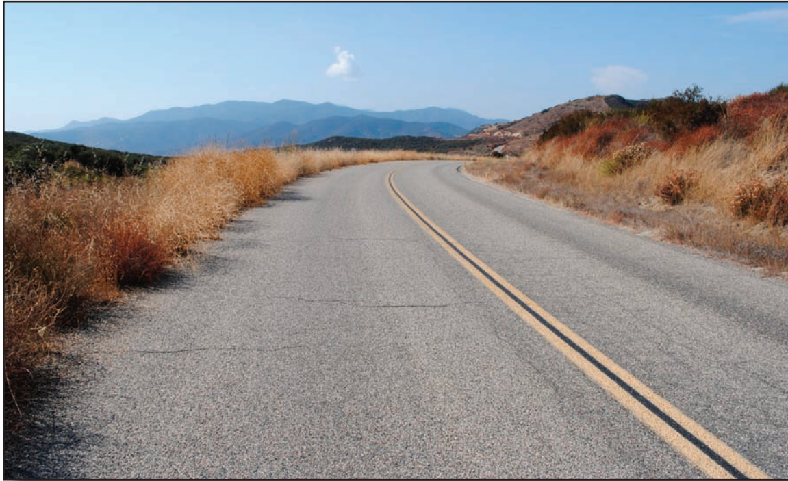
Figure 3—Maintenance level 5 double-lane road with an asphalt surface and grass on the shoulders. Speed limits may be posted as necessary with a Code of Federal Regulations (CFR) order after completion of an engineering study. Grass on shoulders is acceptable and helps with stabilization. Pavement cracking should be monitored so it can be repaired before it has a negative effect on the high level of user comfort and convenience expected on a maintenance level 5 road. Edge markings are not required on a paved road. Ditches are kept clean to facilitate drainage.
