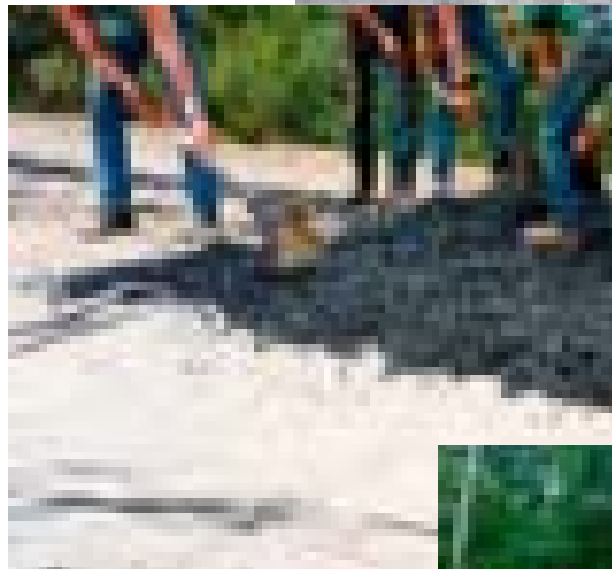
Figure 3.1f— Geosynthetic used immediately beneath asphalt.
