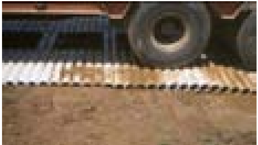
Figure 3.5—Fascine (Mason and Moll 1995).
