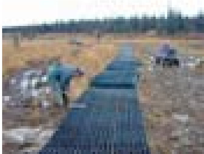
Figure 3.1k— Caribou Lake Trail using Solgrid, intended for minimal visual impact, Alaska, (Kevin Meyer, National Park Service).
