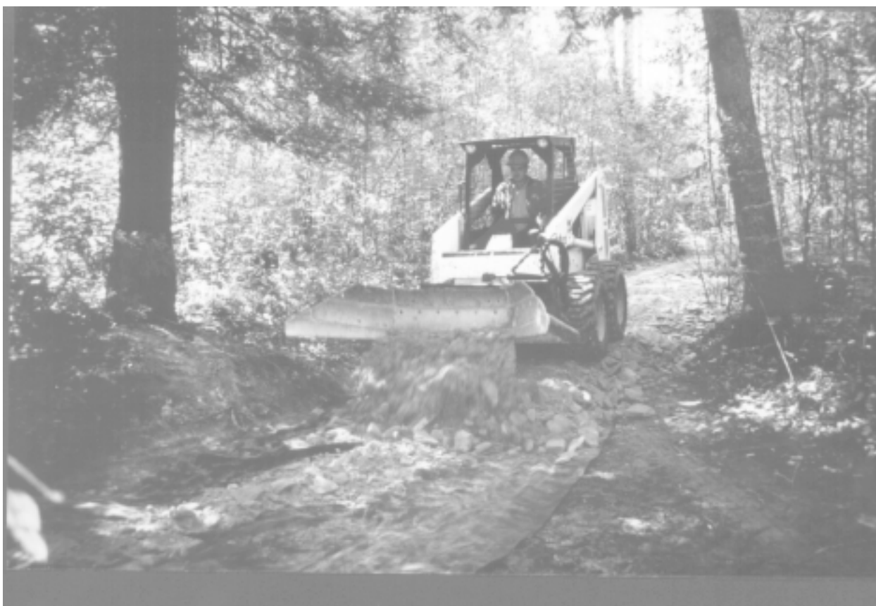
Figure 19A.—Bobcat 763 Skid-Steer loader with a modified blade.
