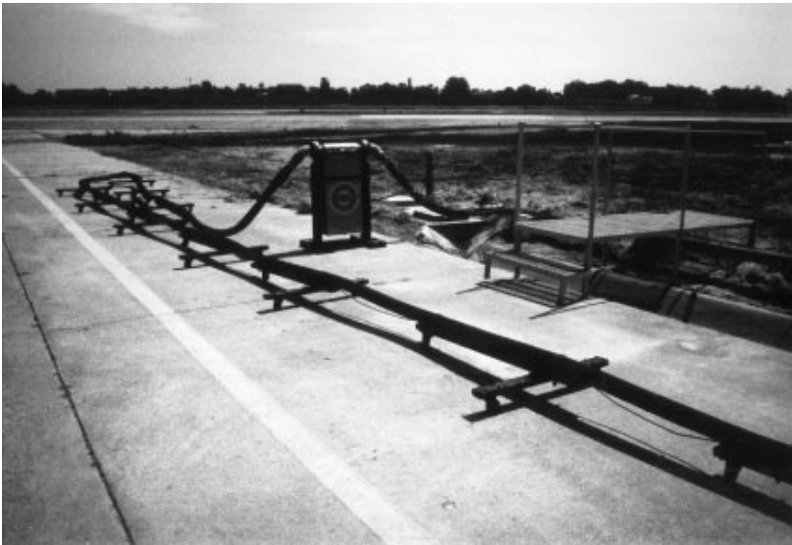
Figure 48. Residues Collection Trench with Sump—Santa Barbara, CA.
