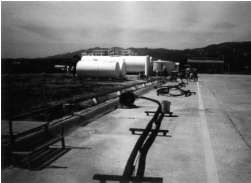
Figure 53. Drainage Trench—Santa Barbara, CA.
