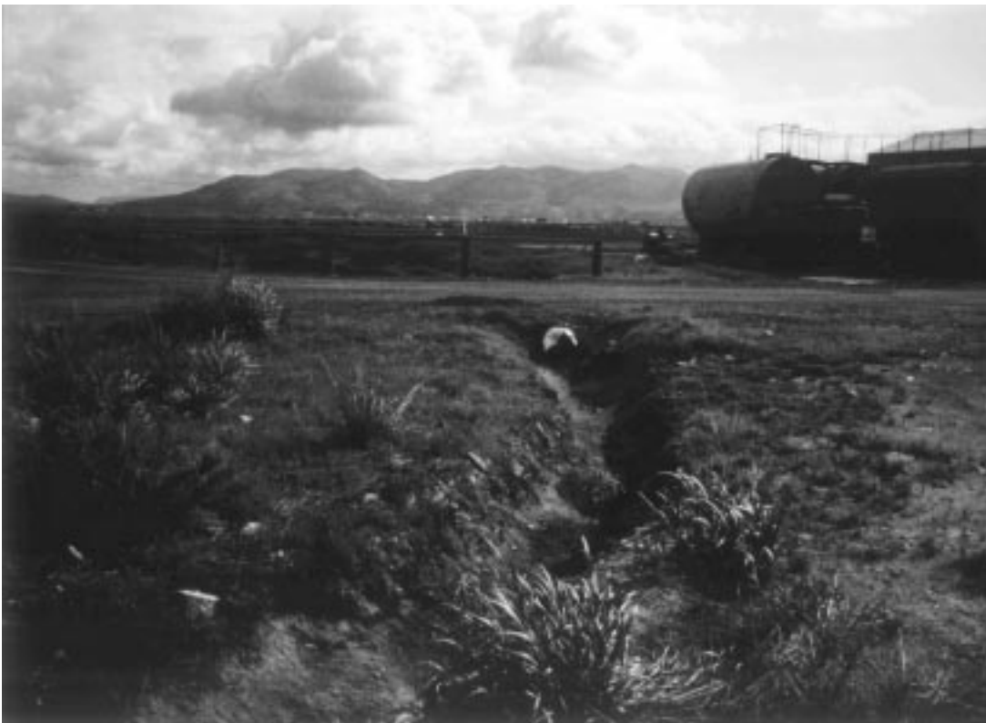
Figure 22. Overflow Culvert and Drainage—Lakeview, OR.
