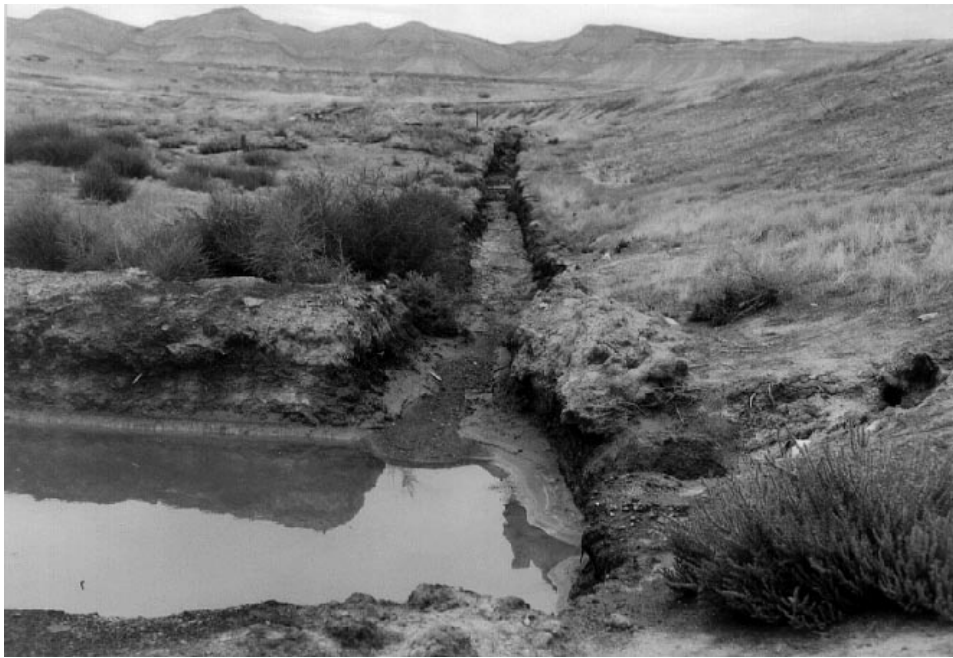
Figure 33. Unlined Drainage Trench—Grand Junction, CO.
