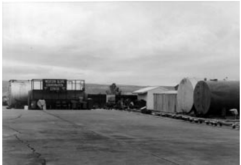
Figure 32. Retardant Storage Tanks—Grand Junction, CO.
