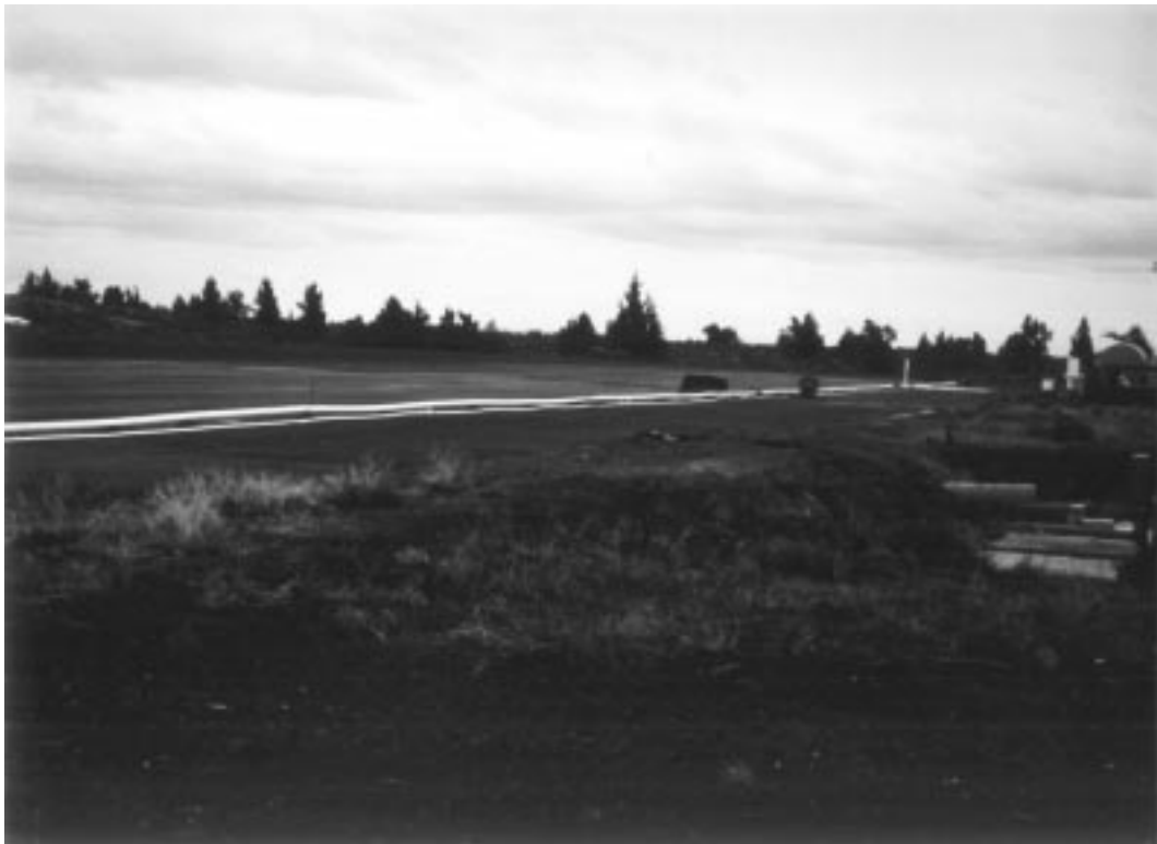
Figure 16B. Runway Drain—Redmond, OR.
