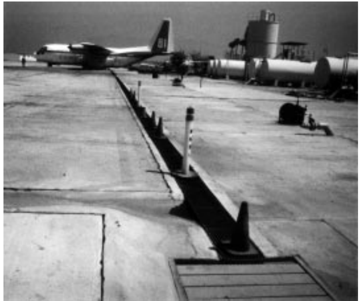
Figure 47. Residues Collection Sump—Hemet, CA.
