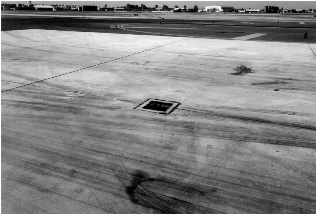
Figure 35. Aircraft Loading Pad Drain—Fresno, CA.
