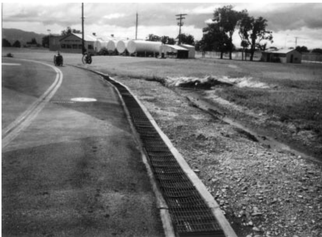
Figures 27 A&B. Loading Ramp Drains—Medford, OR.
