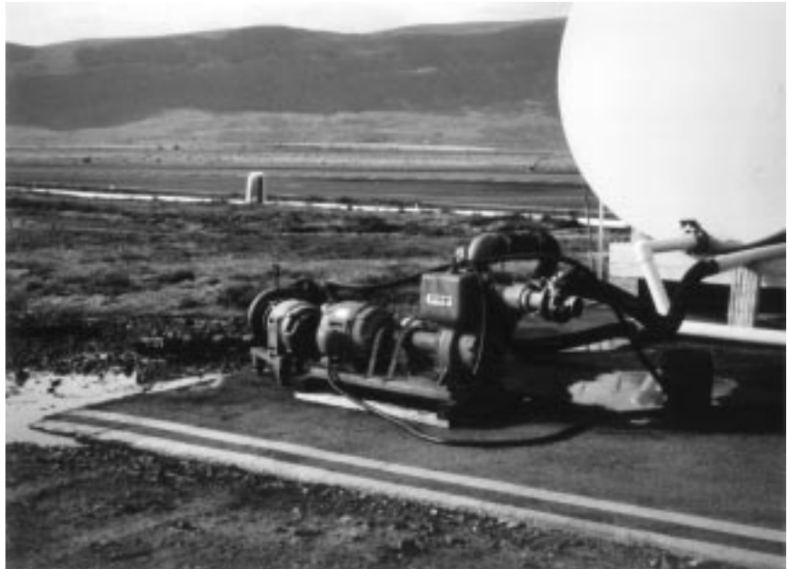
Figure 11. Storage Tank Pad—Wenatchee, WA.
