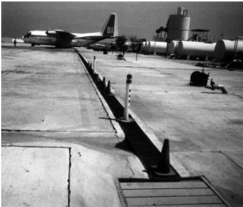
Figure 5. Base Drainage Ditches—Hemet, CA.
