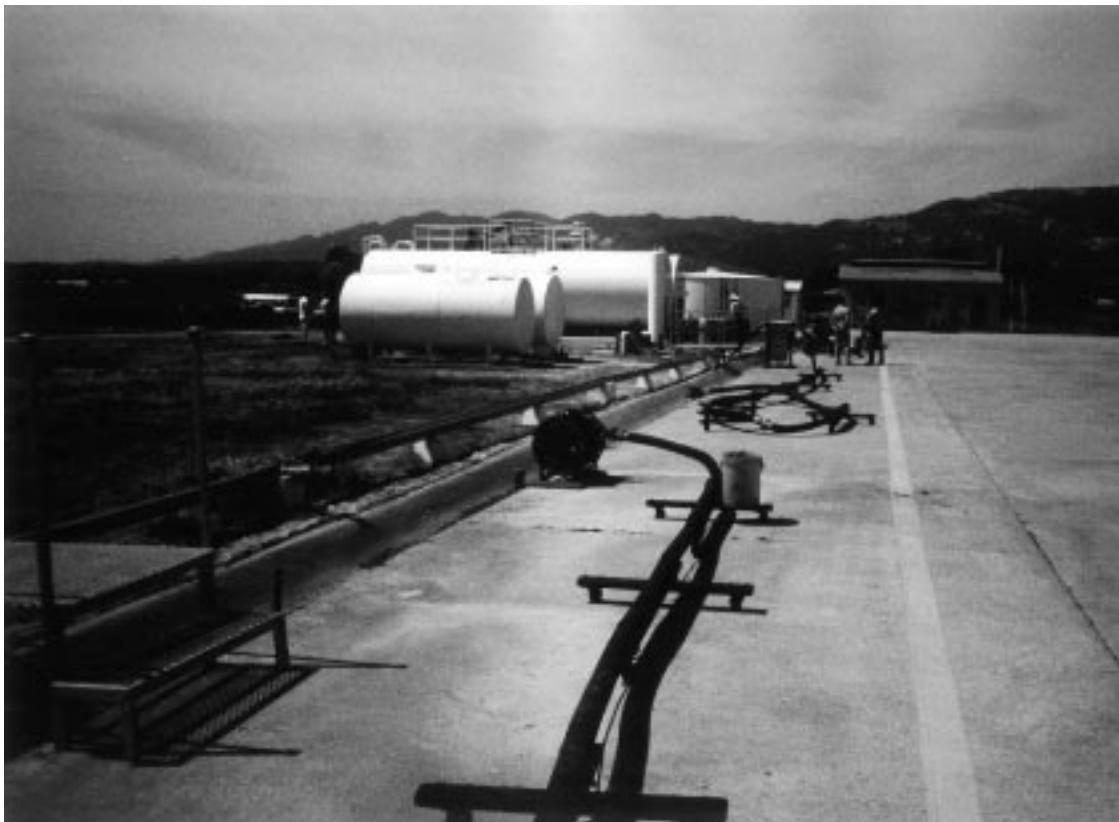
Figure 9. Drainage Trench—Santa Barbara, CA.
