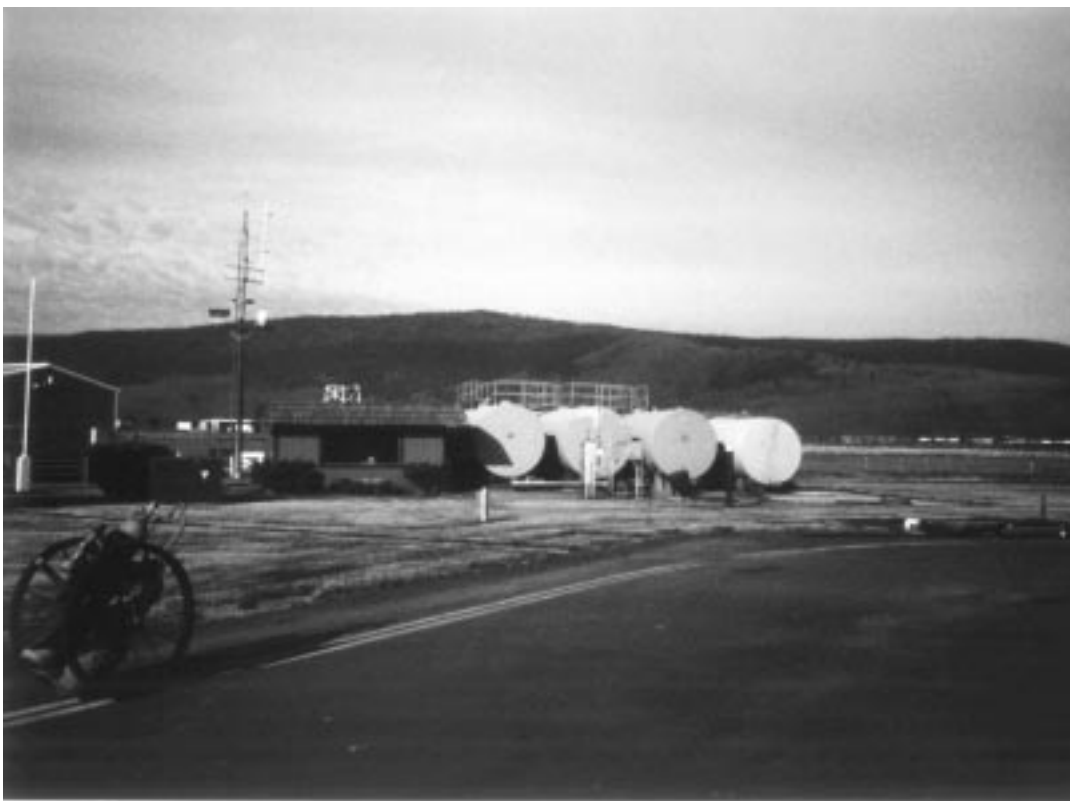
Figure 18. Ramp Drainage—LaGrande, OR.
