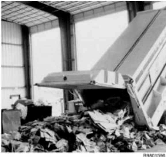
Figure 3. Typical materials recovery facility where recycled resources are sorted and recovered.
