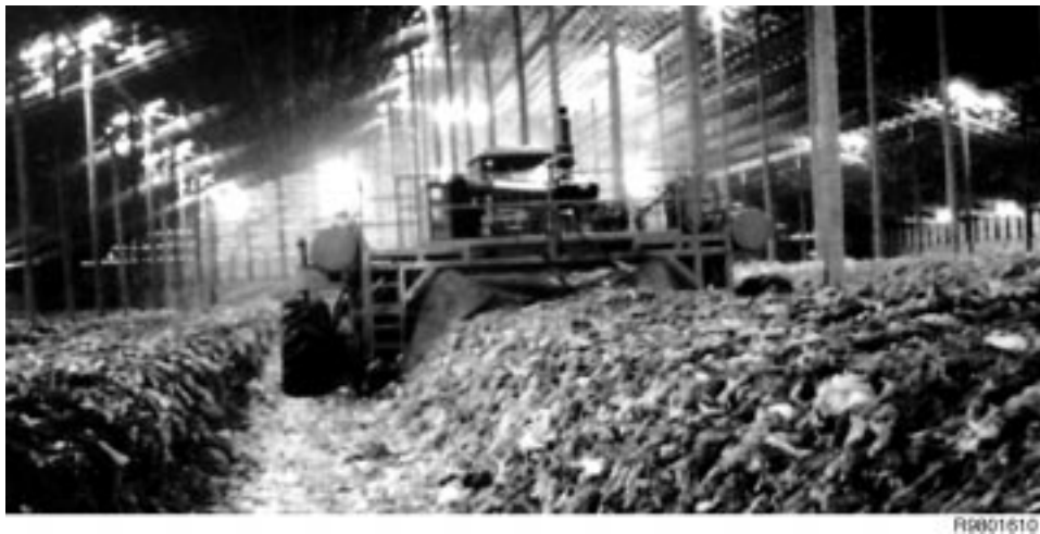
Figure 17. An indoor solid waste composting facility.
