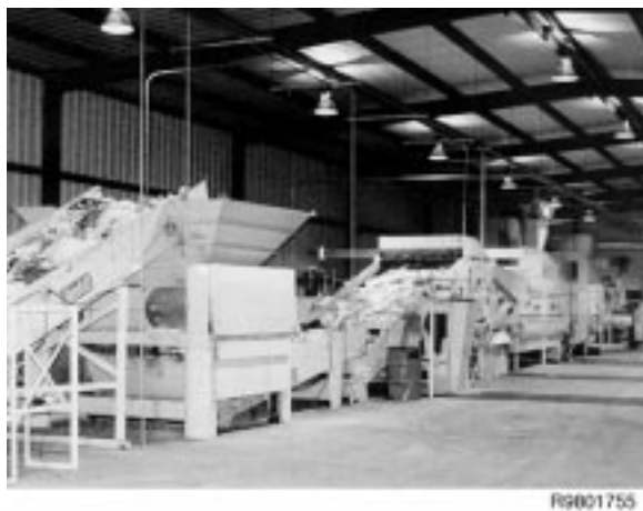
Figure A58. MRF recycling two line system that can process up to 200 tons-per-day with automatic aluminum, steel, ferrous metals, stainless brass and non ferrous, compost and paper separation. By Lundell Manufacturing Company Cherokee, Iowa (712) 225-5181 Fax: (712) 225-5185
