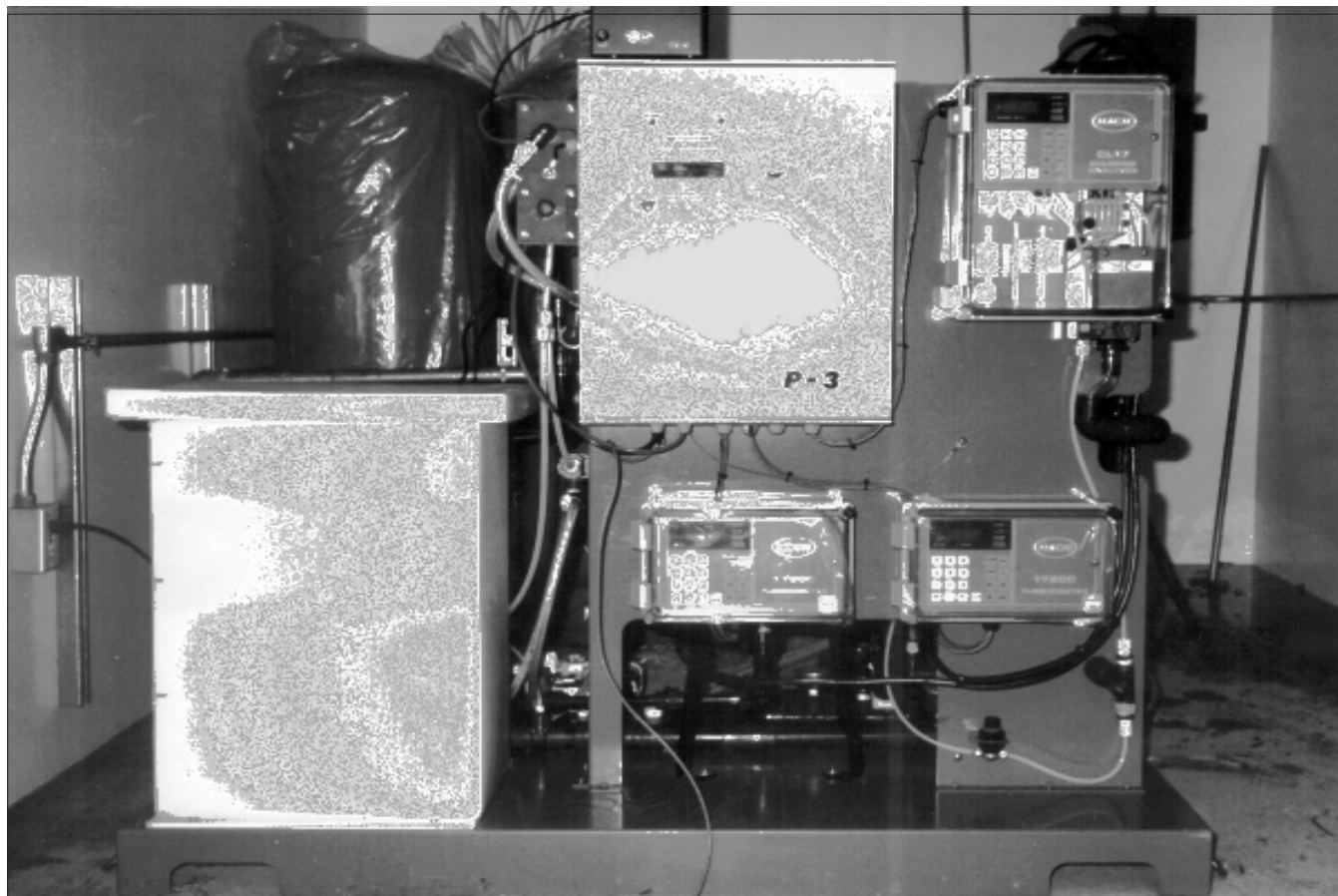
Figure 1.—The MIOX P-3 installed at Priest Lake campground, Idaho.
