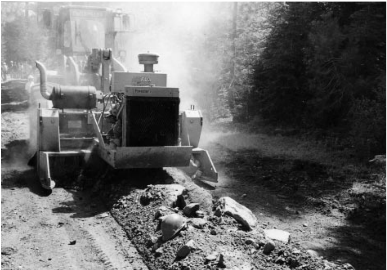
Figure 1—Forester C-2000 Road Crusher.
