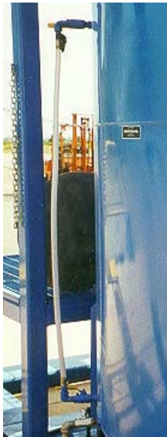
Figure 11—Mixer tank fluid level indicator (sight gage).
