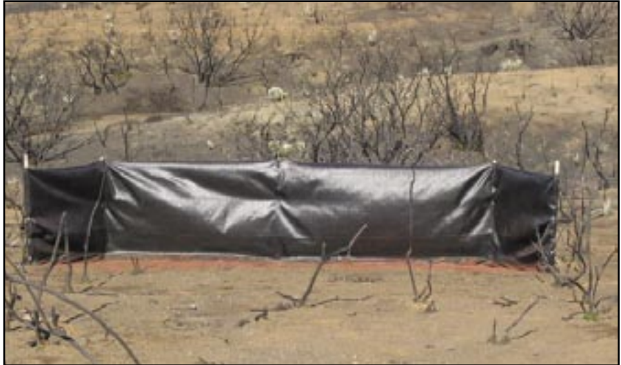
Figure 33—A recently installed silt fence.
