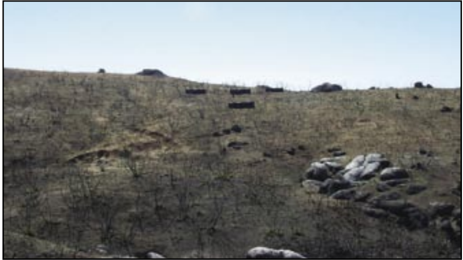
Figure 35—Silt fences are effective at trapping sediment but require inspection and maintenance. Silt fences should be removed once the area has stabilized.
