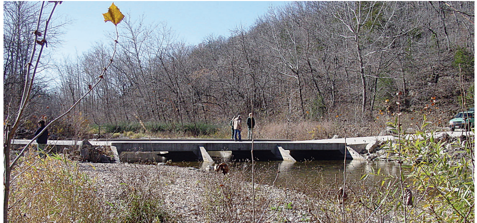
Figure 1.7—High-VAR ford composed of three box culverts, Mark Twain National Forest, Missouri.
