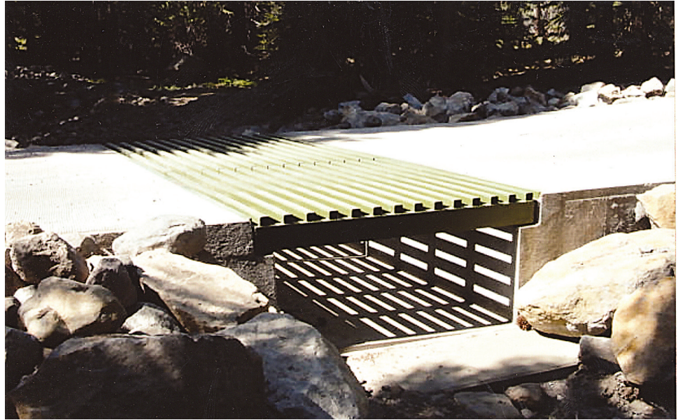
Figure A84. Close up of grate-top vented ford.
