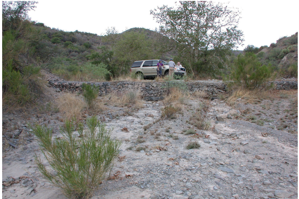
Figure A21. This jersey barrier-gabion ford on the 7-Springs Road on the Tonto replaced a bridge washed out in a flood.
