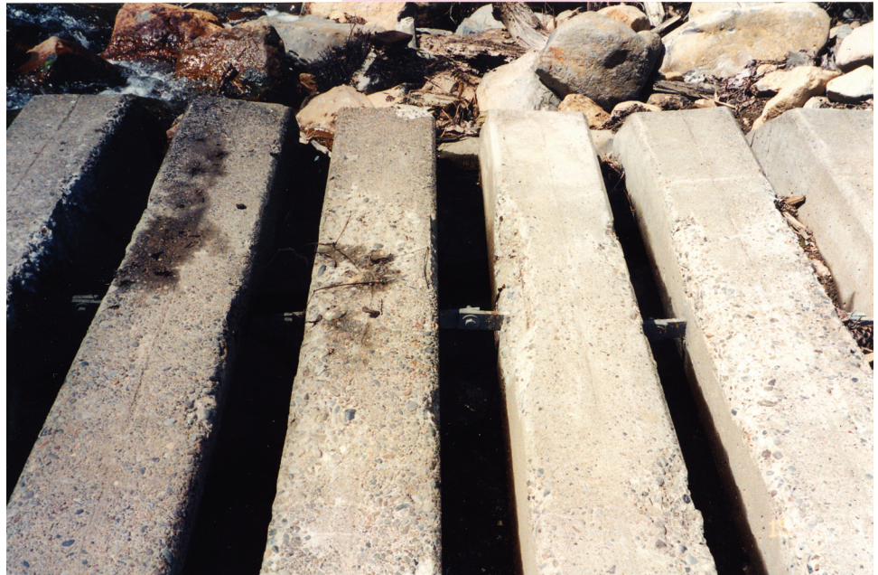
Figure A24. Detail of planks and metal brackets.
