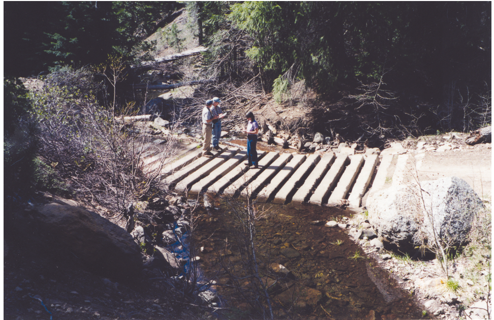
Figure A23. Looking downstream: ford is just above a tributary junction where an old diversion structure blew out and caused streambed to degrade.
