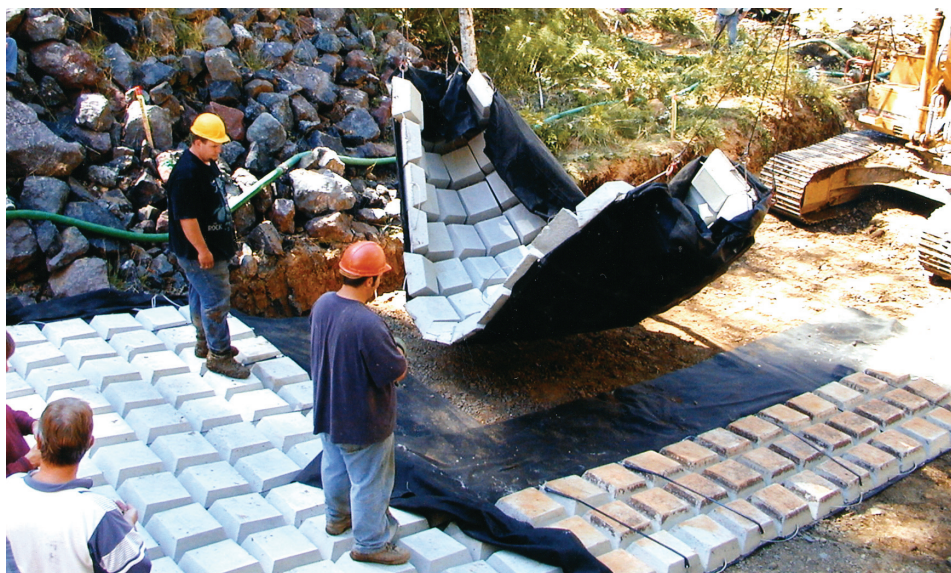
Figure A30. An excavator installs the mats with geotextile backing.
