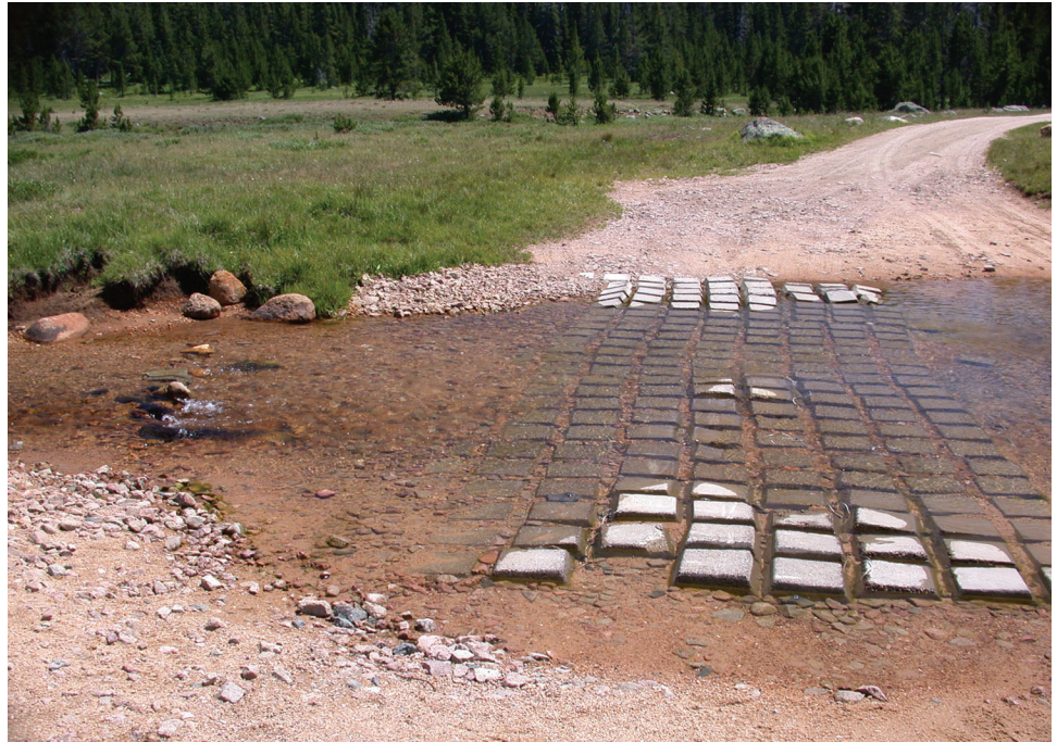
Figure A32. East Fork South Tongue River cable concrete block mat crossing. Note tilted blocks, exposed cables, and short mat length. Traffic is driving around the mat and the river has outflanked it.
