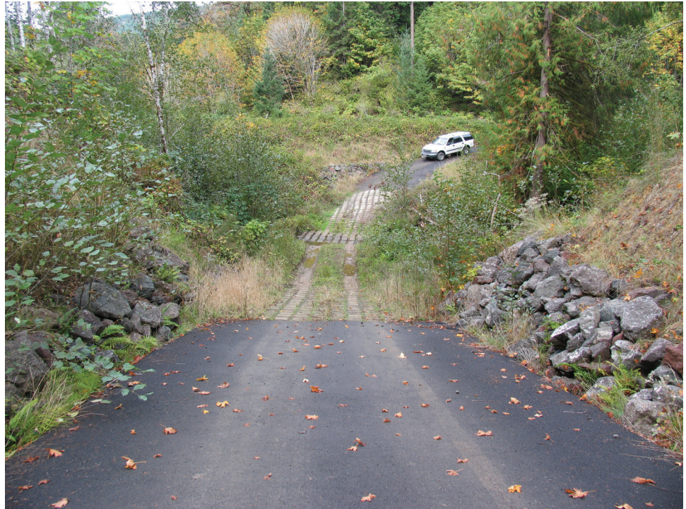
Figure A27. Fitzpatrick cable concrete mat ford.
