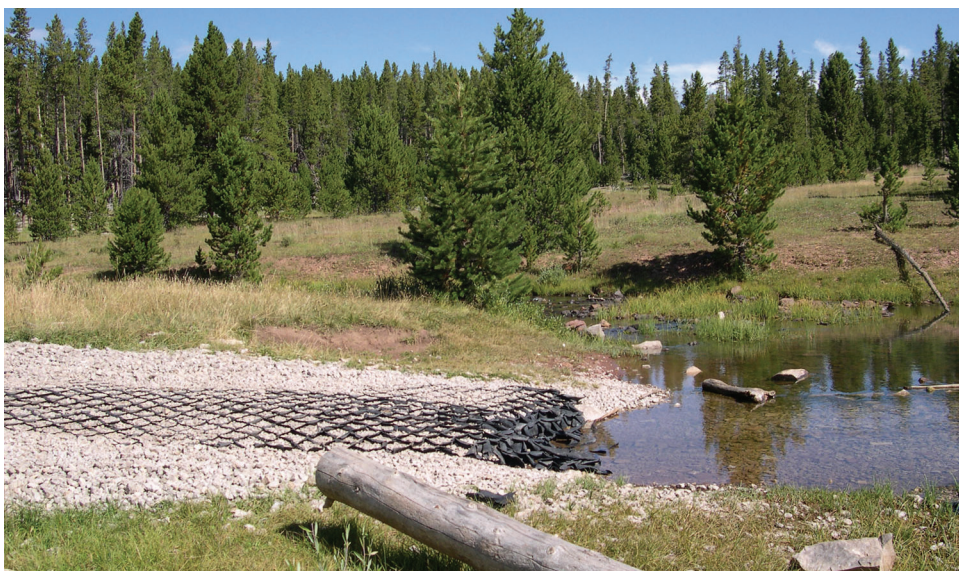
Figure A41. Looking upstream at erosion of one side of the ford in August 2004, 3 years after construction. Probably tire action and high flows have combined to pluck material out of the cells or undermine them. The ford is still intact and the geocells are covered by native bed material in the active channel.
