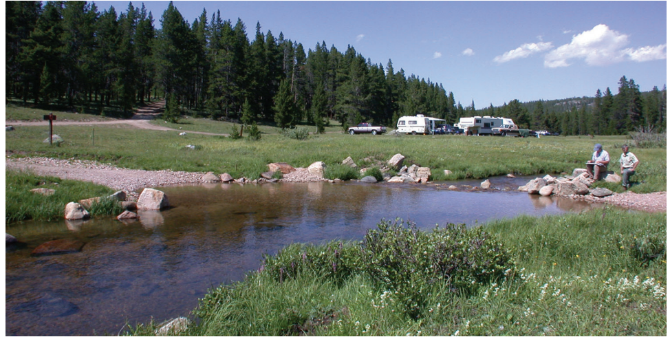
Figure A38. Soil compression on the approaches to the ford causes the stream to widen and lowers the elevation of the ends of the Geoweb mat. Currently the geocell mat protects only part of the crossing during high flows.
